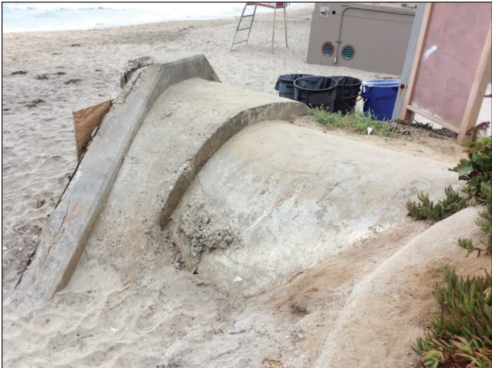
Figure 4. Outfall and diversion structure; View facing northwest.
