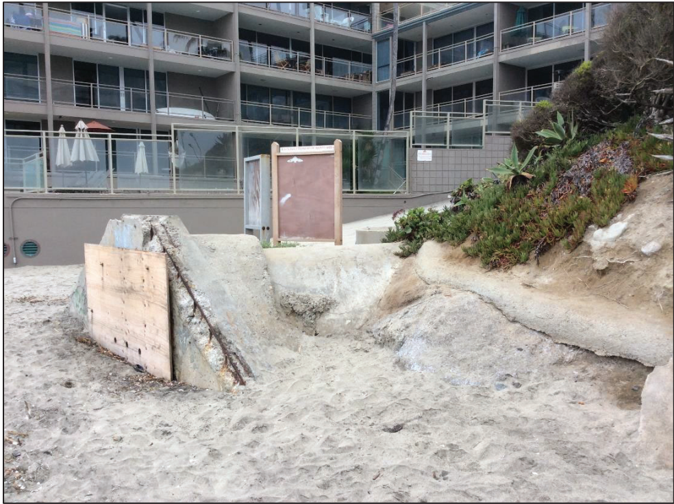
Figure 3. Outfall and diversion structure; View facing northeast.
