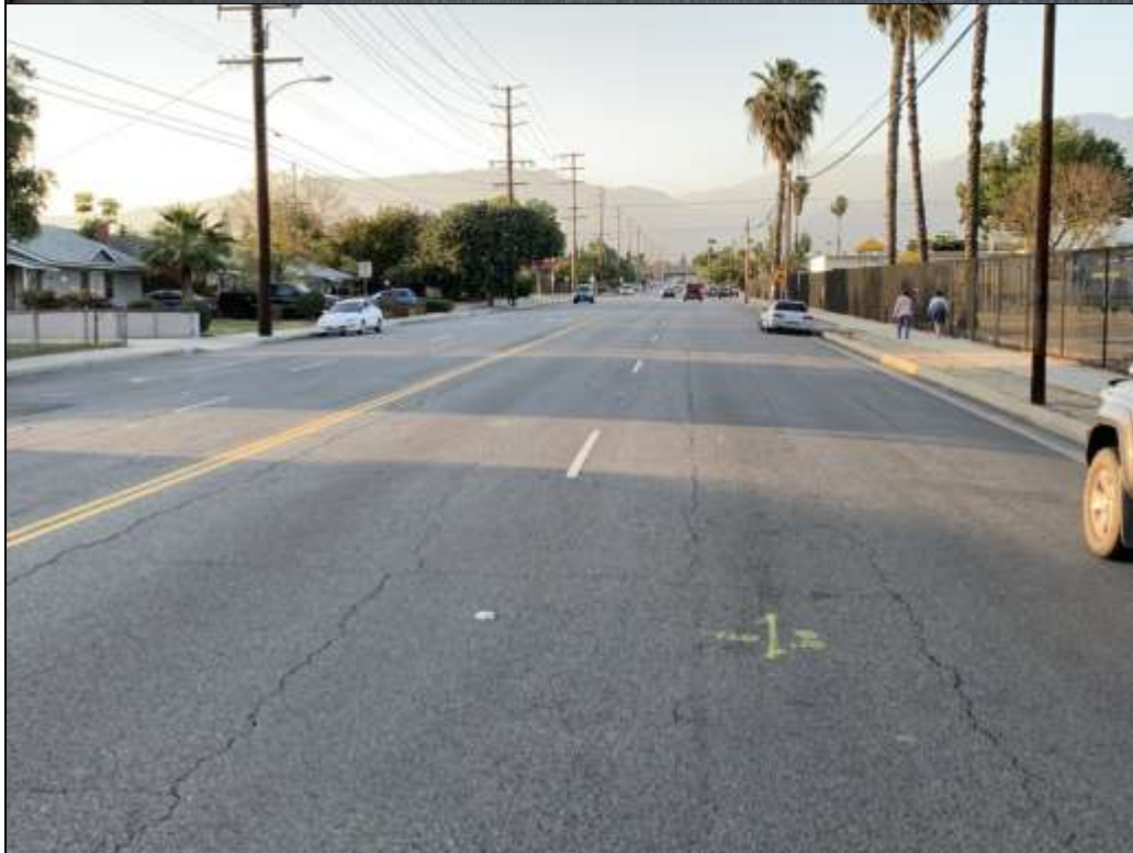
Photo 6. Looking north towards Well 33 facility down pipeline alignment along east side of Benson Ave at the intersection with Princeton St.
