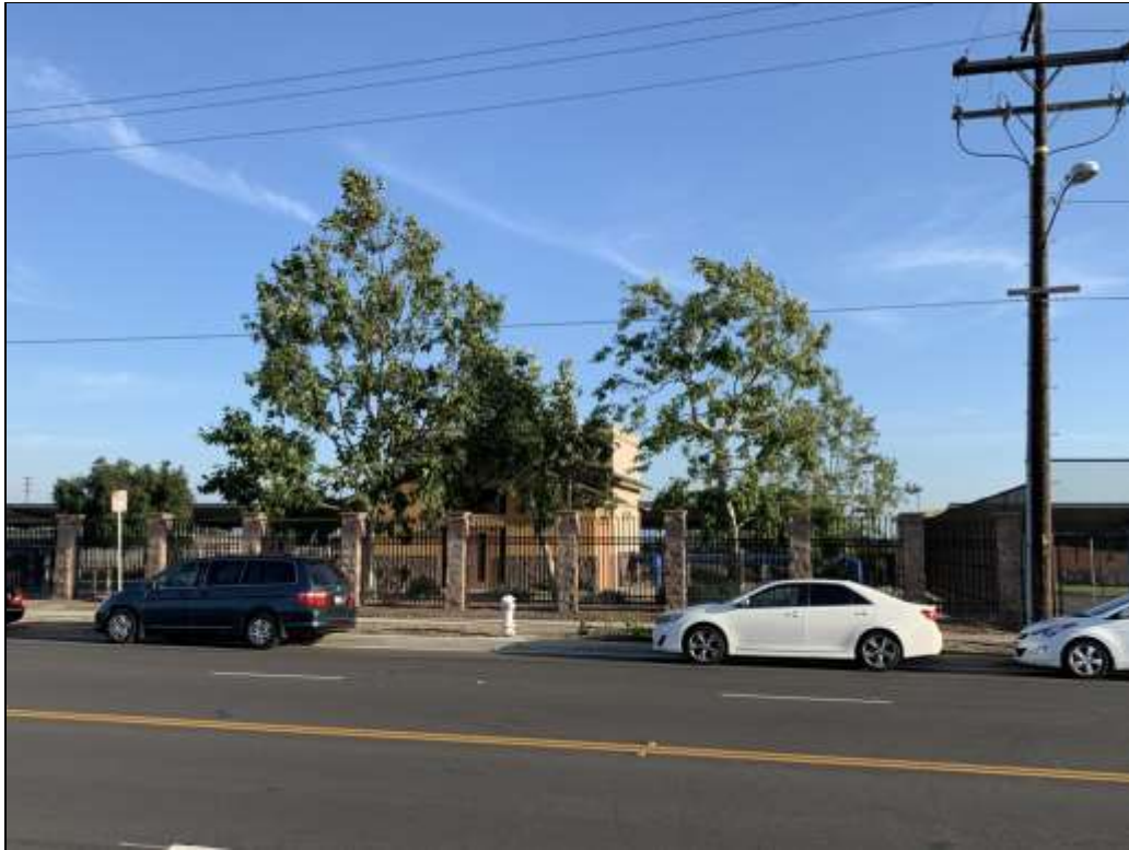
Photo 7. Looking south across San Bernardino St. at Well 30 facility.
