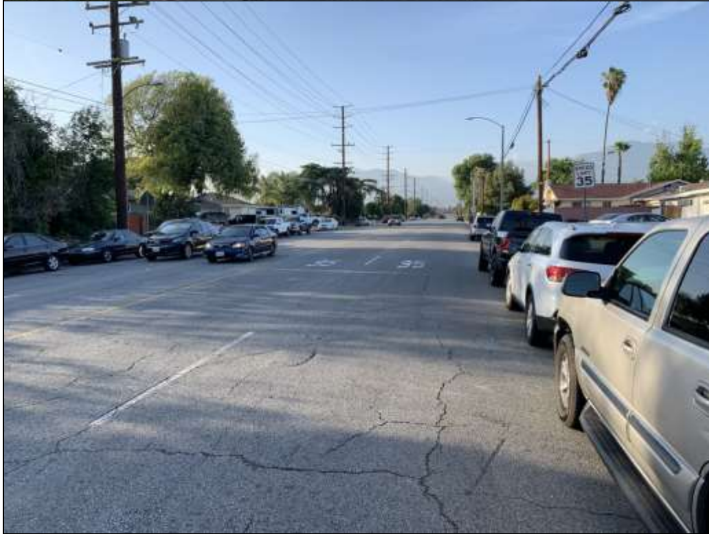
Photo 12. Looking north down Benson Ave. along pipeline alignment towards Well 33 facility from the intersection with San Bernardino St.
