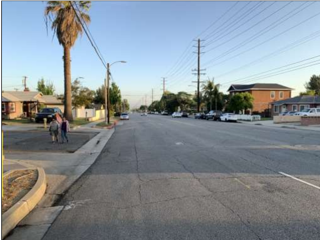
Photo 5. Looking south down pipeline alignment along east side of Benson Ave at the intersection with Princeton St.
