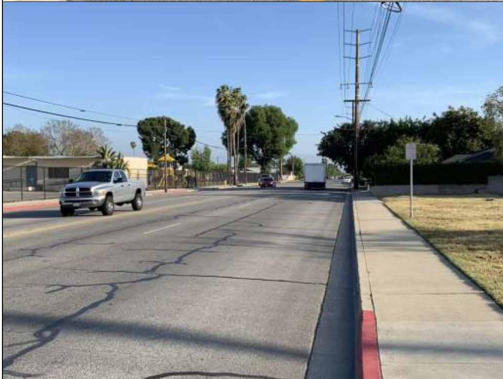
Photo 4. Looking south down west side of Benson Ave. south of Palo Verde St.
