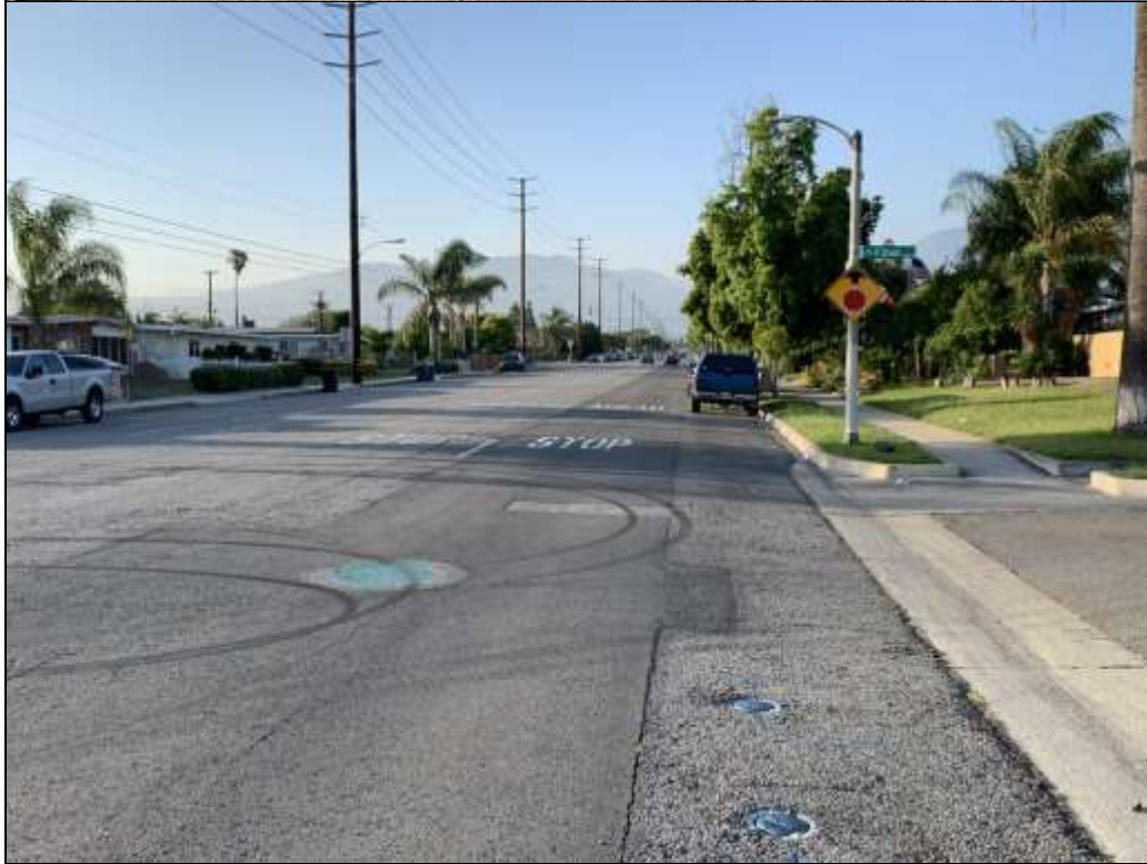
Photo 14. Looking north down the east side of Benson Ave. along pipeline alignment from the intersection of H St.
