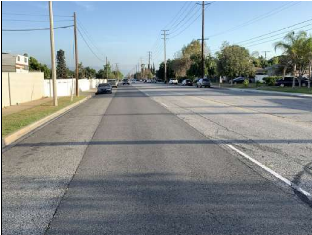
Photo 15. Looking south down the east side of Benson Ave. along pipeline alignment from the intersection of H St. towards Well 32 facility.
