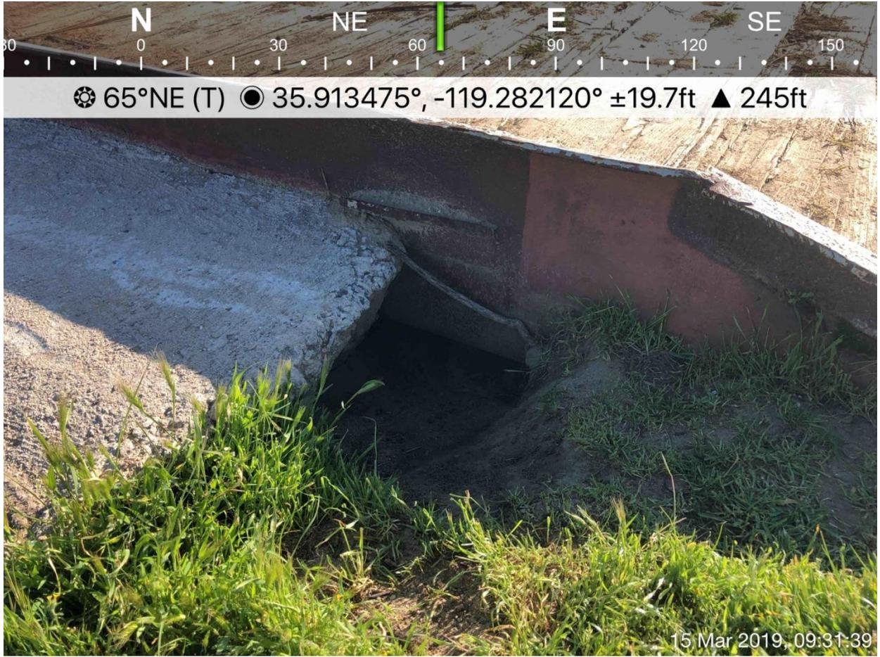
Photograph 11: Burrows were observed beneath the Deer Creek check structure bridge.
