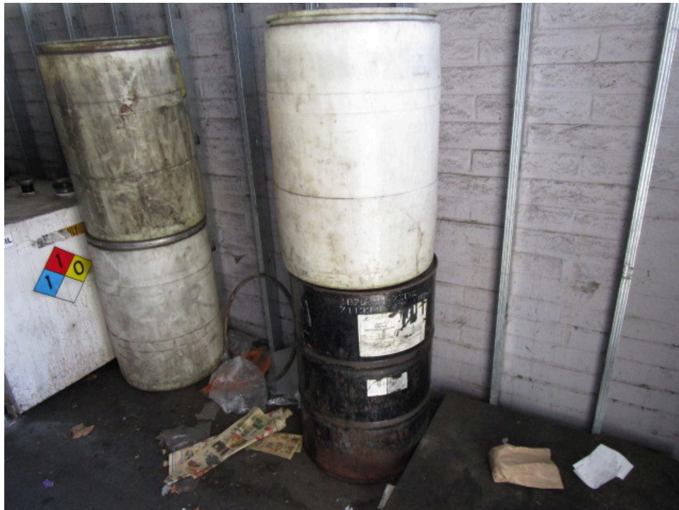
14. Empty drums and an anti-freeze drum in the enclosure on the southern side of the building
