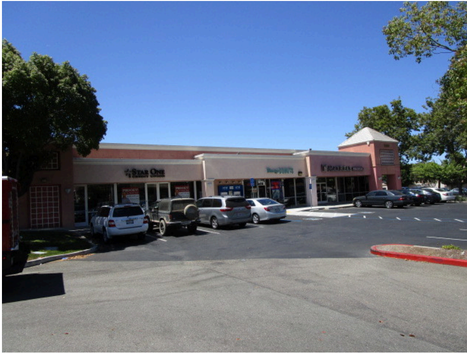
41. Multi-tenant retail building (10991 North De Anza Boulevard) adjacent to the north
