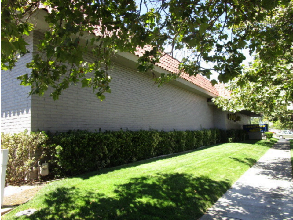
5. Eastern side of the subject property building
