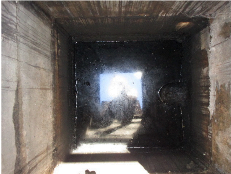
7. Interior of the clarifier
