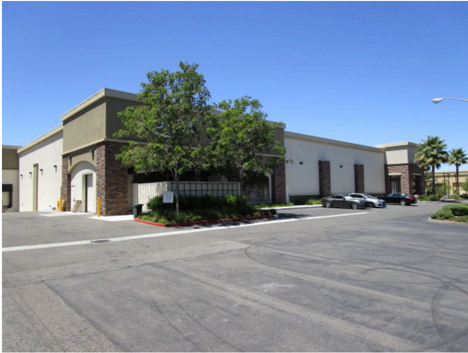
39. Ulta Beauty (20580 Homestead Road) adjacent to the west
