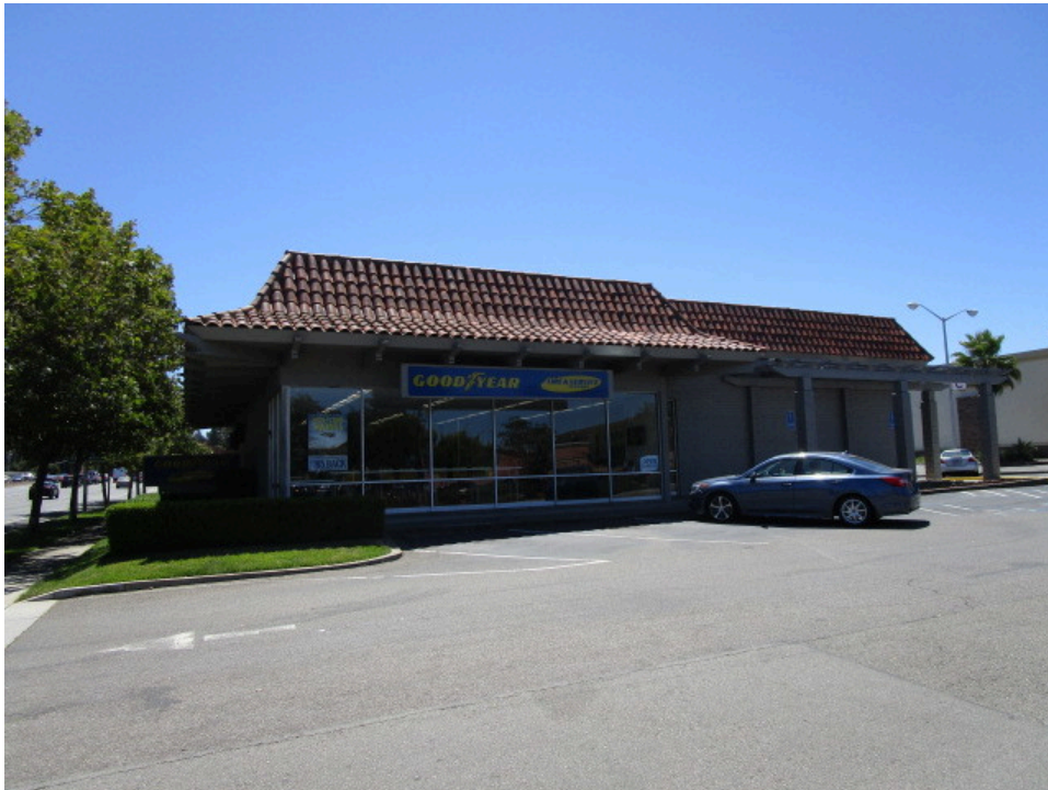
2. Northern side of the subject property building
