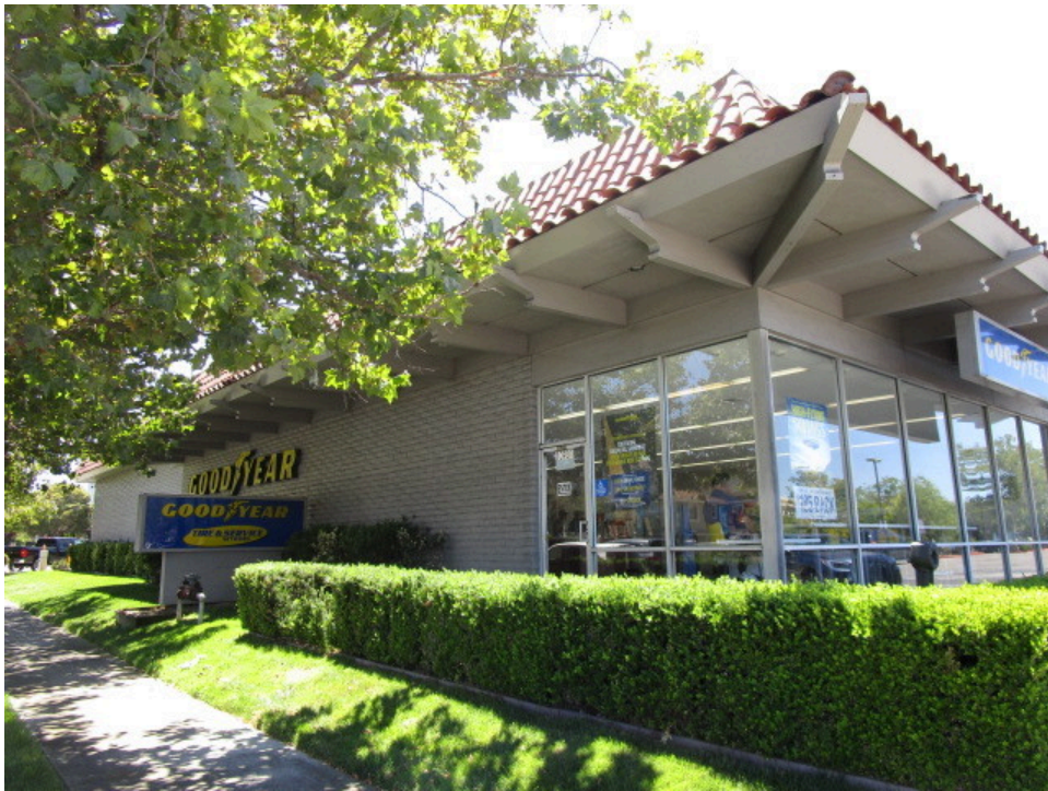
4. Eastern side of the subject property building
