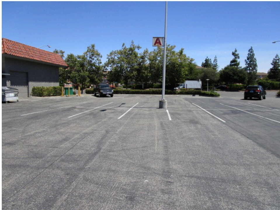
8. Asphalt-paved parking/drive area on the subject property
