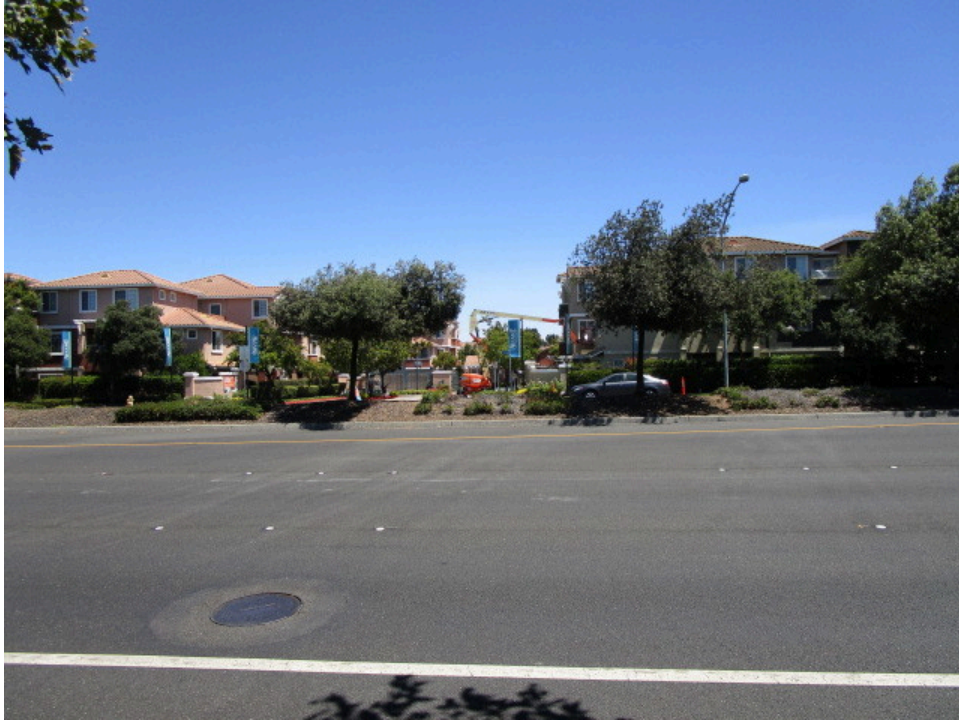
43. Aviare Apartments (20415 Via Paviso) adjacent to the east
