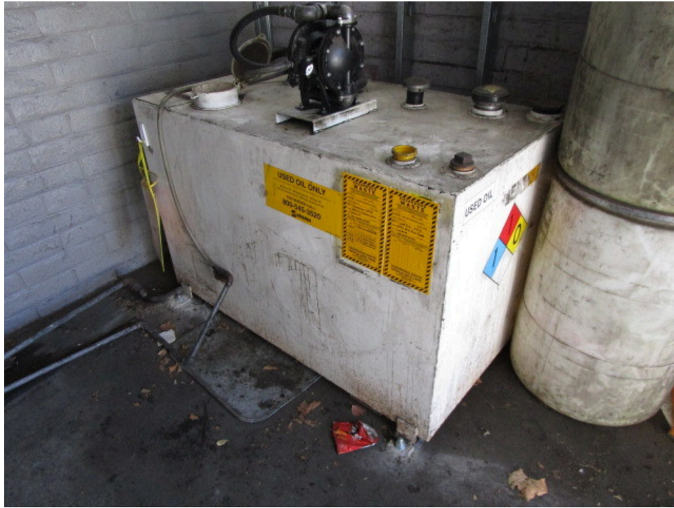
13. Waste oil AST in the enclosure on the southern side of the building
