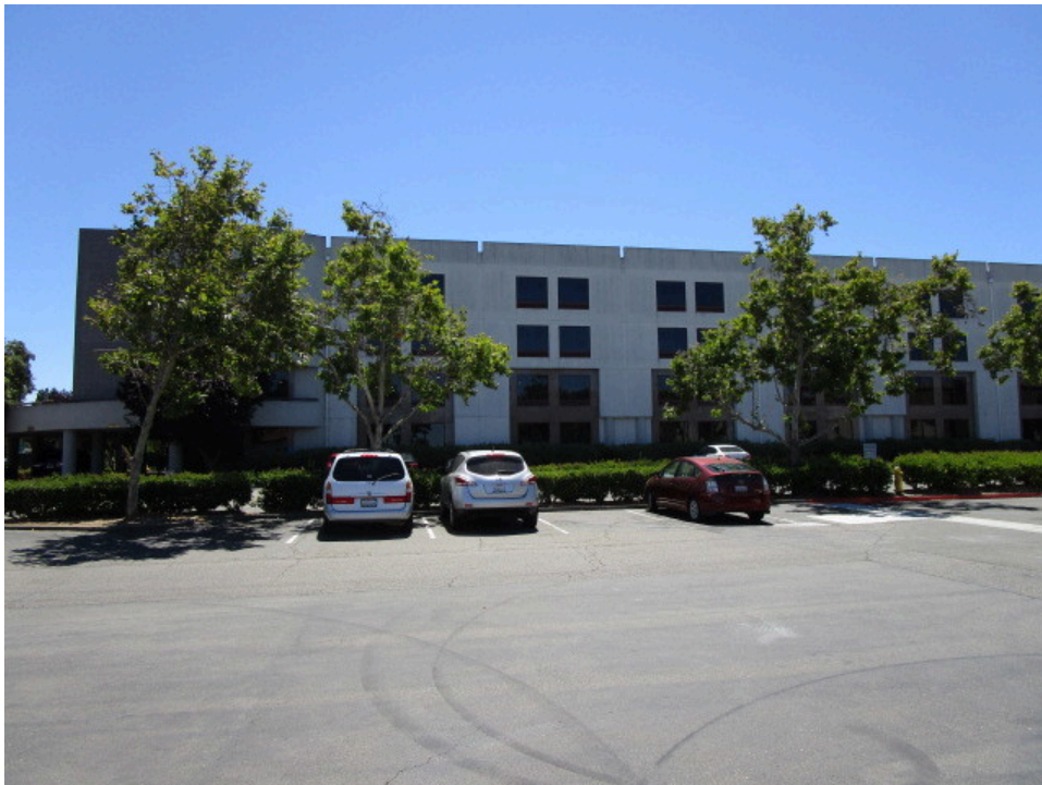
40. Cupertino Hotel (10889 North De Anza Boulevard) adjacent to the south
