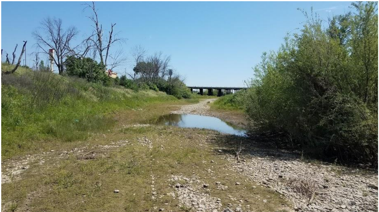
Figure 2. A view south along the main channel toward Antelope Blvd. Photo date: April 26, 2018.
