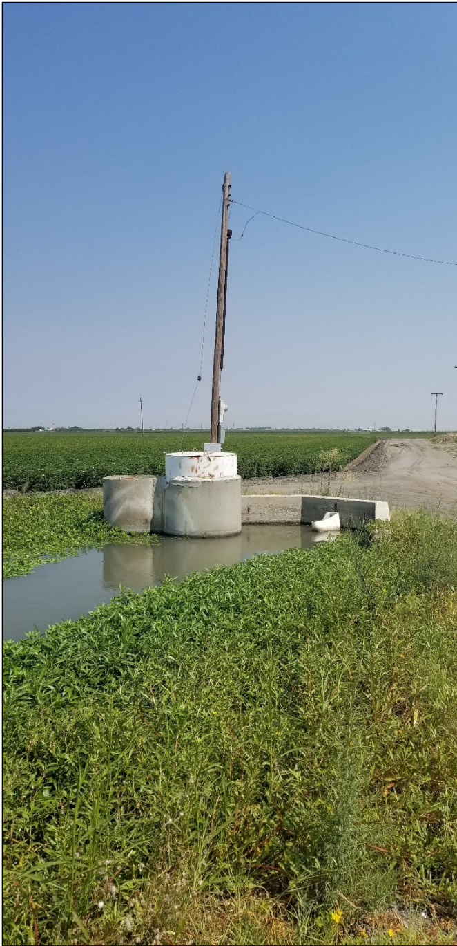
Concrete culvert at Sonoma Avenue, looking northwest.
