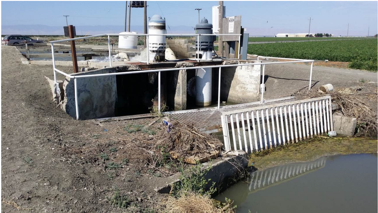
Photo 2: Lift station to be replaced.
