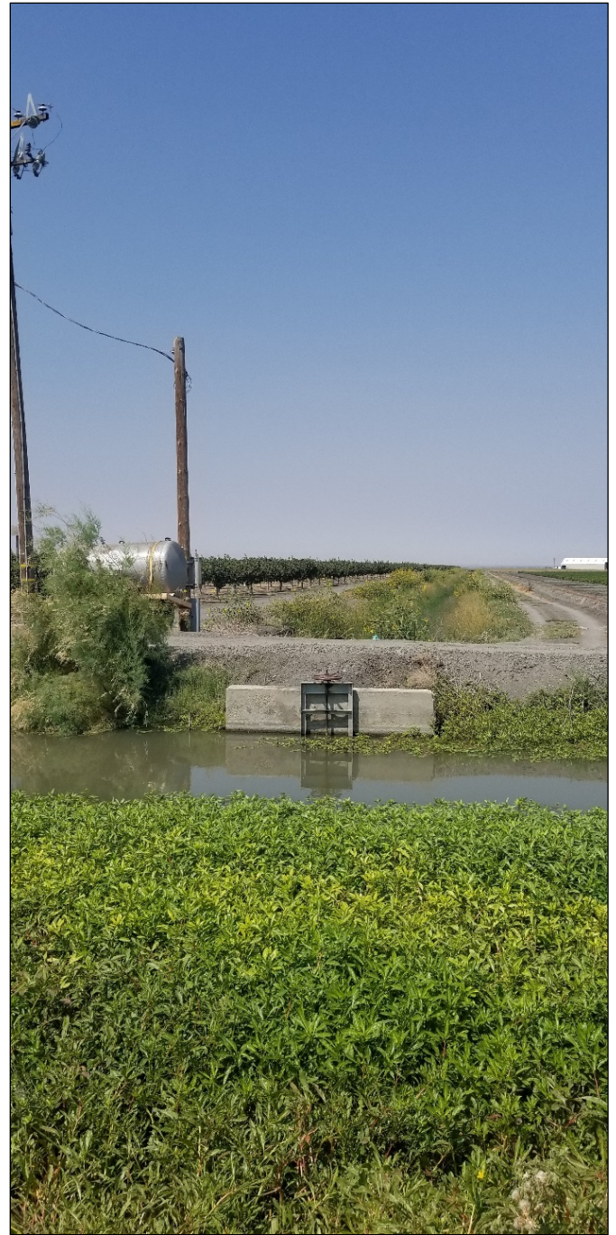
TID Slough Canal and turnout, looking west.
