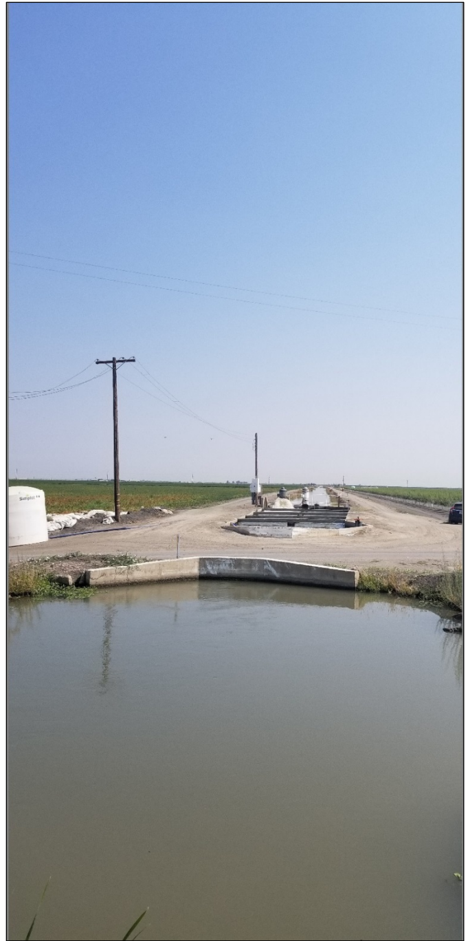
Concrete culvert under Parlier Avenue, looking north.
