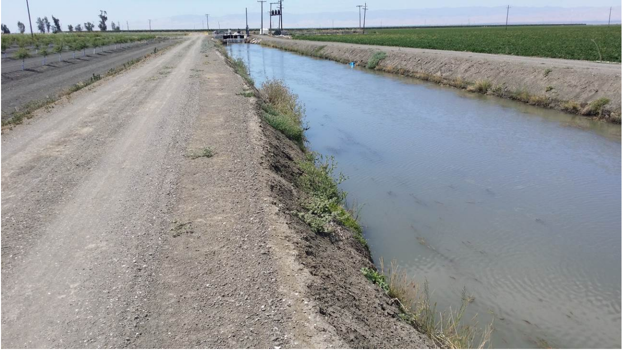
Photo 5: View of the project site from north end of site. Existing lift station in the distance.
