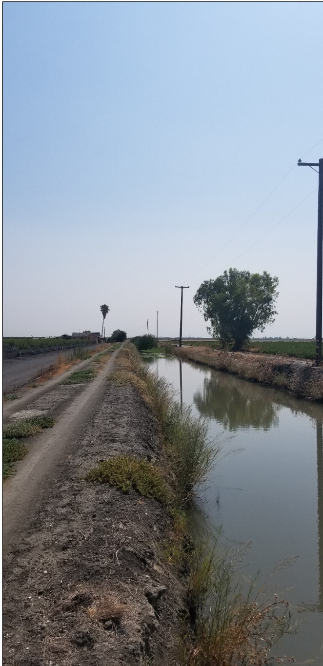
TID Slough Canal, eastern branch north of Parlier Avenue, looking east.
