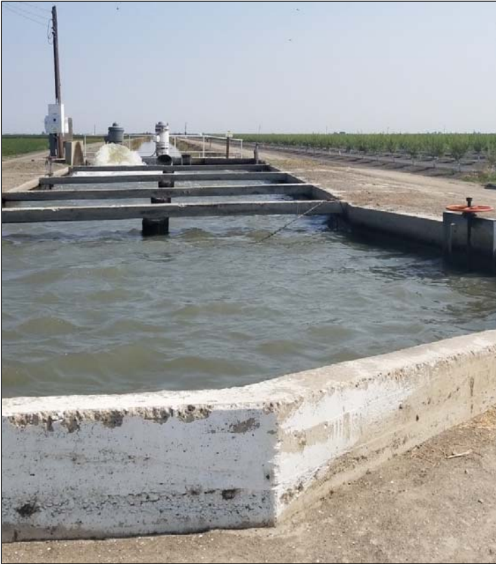
Figure 4-3 Slough Canal showing vertical lift pump system, concrete lining, and turnouts, facing north.
