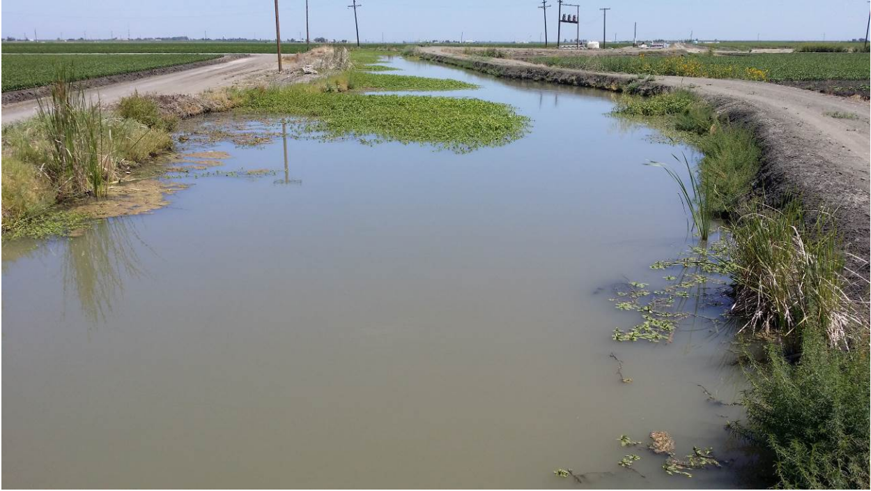
Photo 3: View of project site south of Parlier Ave.
