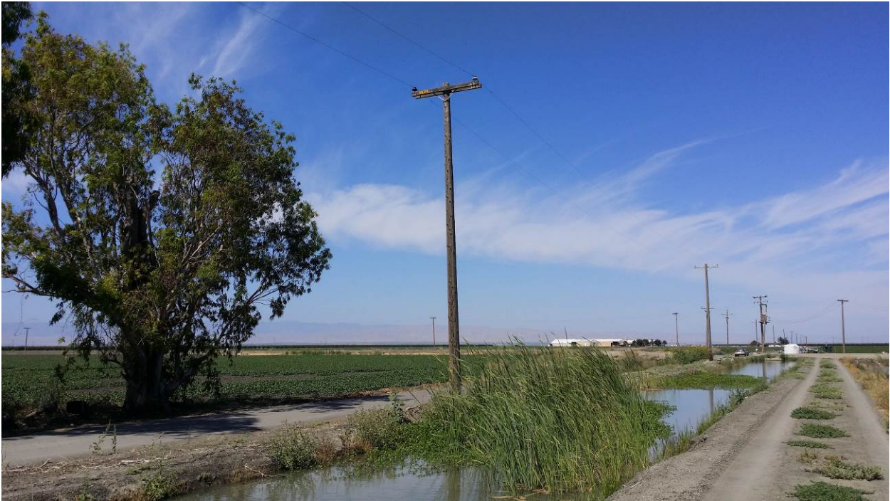
Photo 6: View of the project site from east end of the site looking down a lateral canal toward Slough Canal. Swainson’s hawk nest in eucalyptus tree to left.
