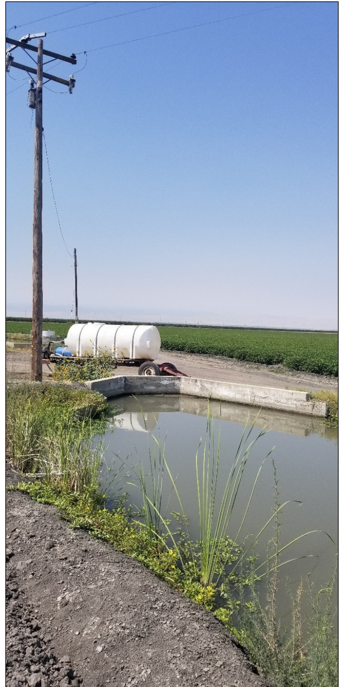
Concrete culvert at Sonoma Avenue, looking southwest.
