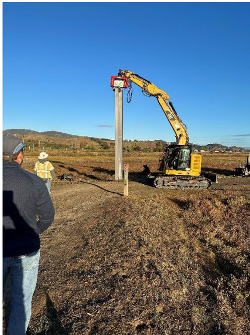
Photo 2: Excavator preparing to install a 20' sheet pile.
