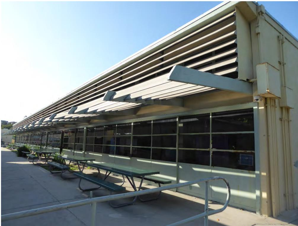
Figure 35. The south façade of Building E, showing metal louvers, pergola, and sliding glass windows and doors.
