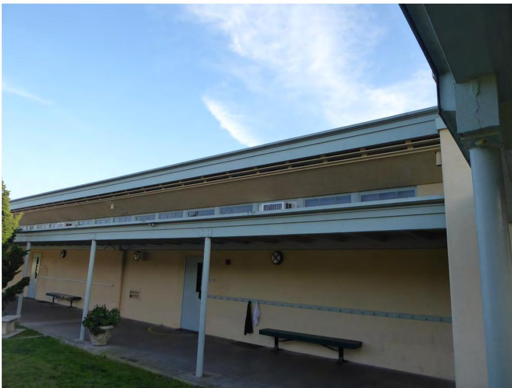
Figure 42. The covered flat canopy and clerestory windows at the north façade of Building G.
