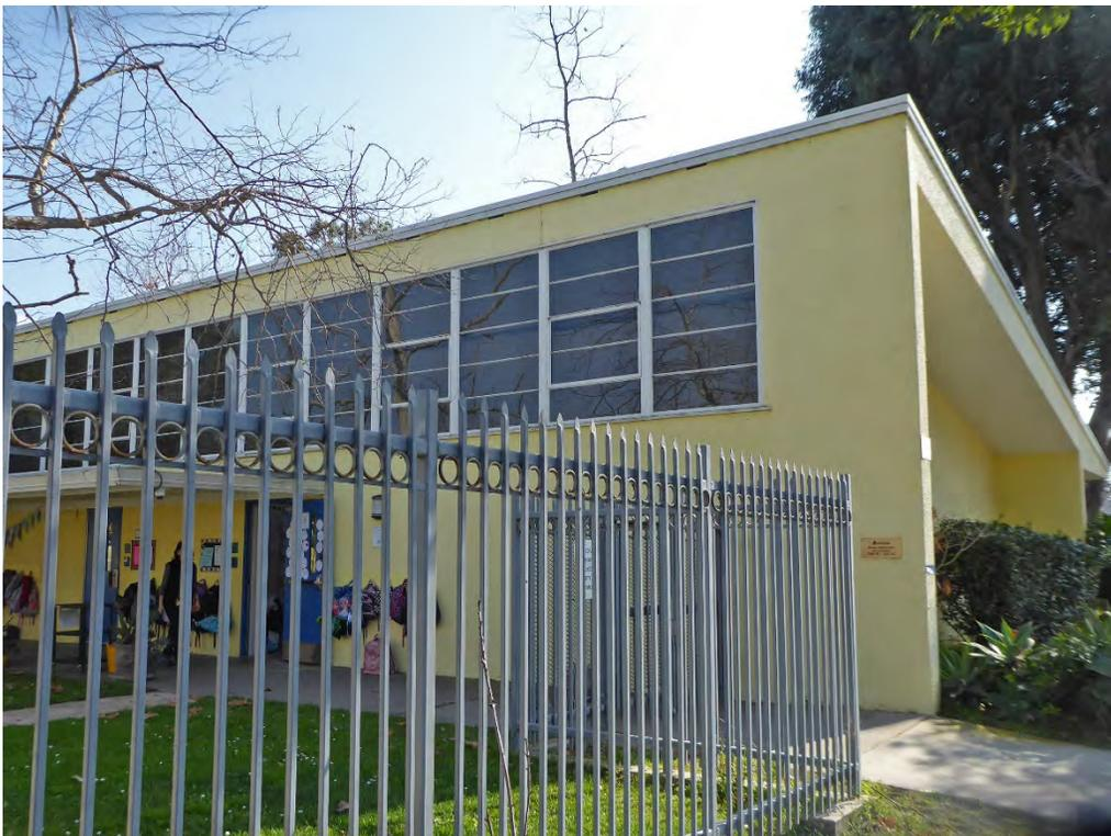
Figure 73. Pacific Elementary School. Detail view of a typical classroom building showing clerestory windows and steep shed roof.
