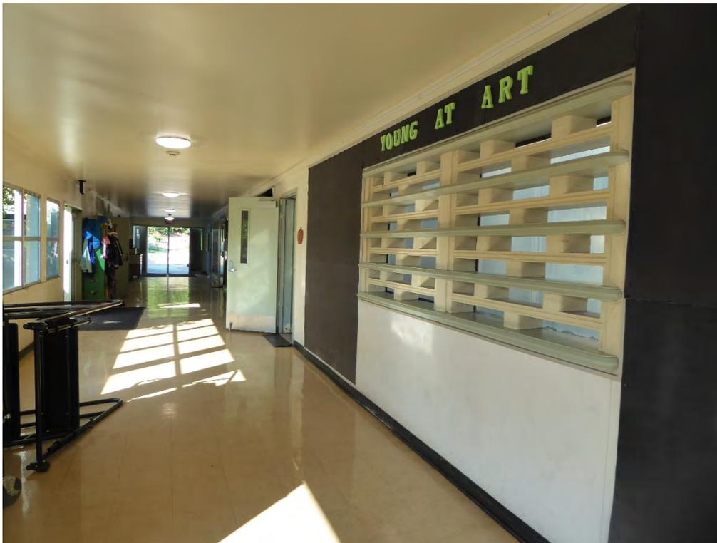
Figure 31. View toward the northeast of the corridor in Building B showing the concrete grille, a design motif used throughout the campus.
