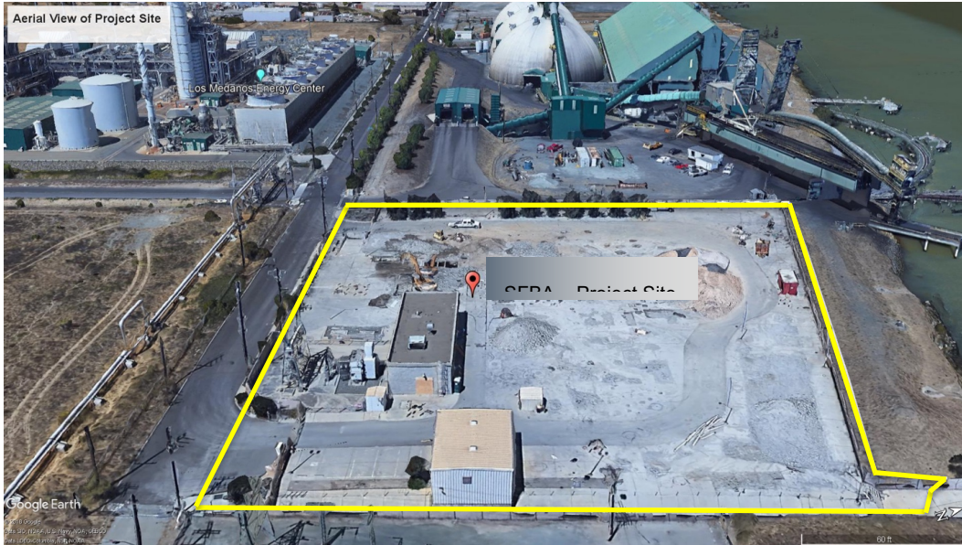
Figure 2 View of Project Site looking west down 3 rd Street.
