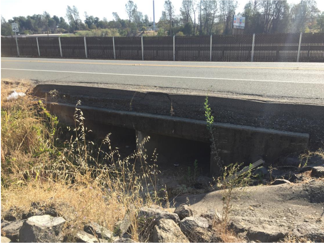
Box culvert under Cascade Boulevard
