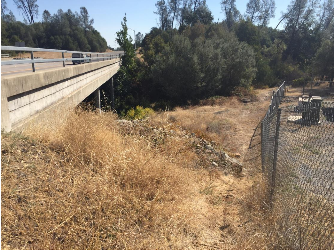
South side of Pine Grove Avenue bridge over Churn Creek
