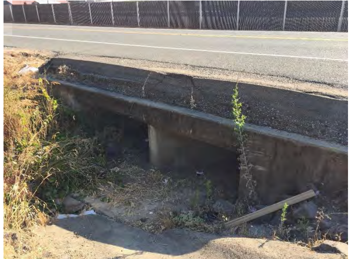
Photo 3.3-1. Box culvert under Cascade Boulevard.
