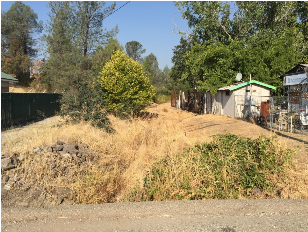
Drainage ditch west of the Cascade Boulevard box culvert
