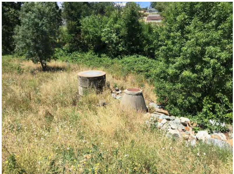
Photo 3.3-8. LS5 Diversion and Overflow Manholes, facing southwest toward Salt Creek.
