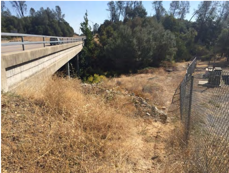
Photo 3.3-6. Pine Grove Bridge over Churn Creek, facing northeast.
