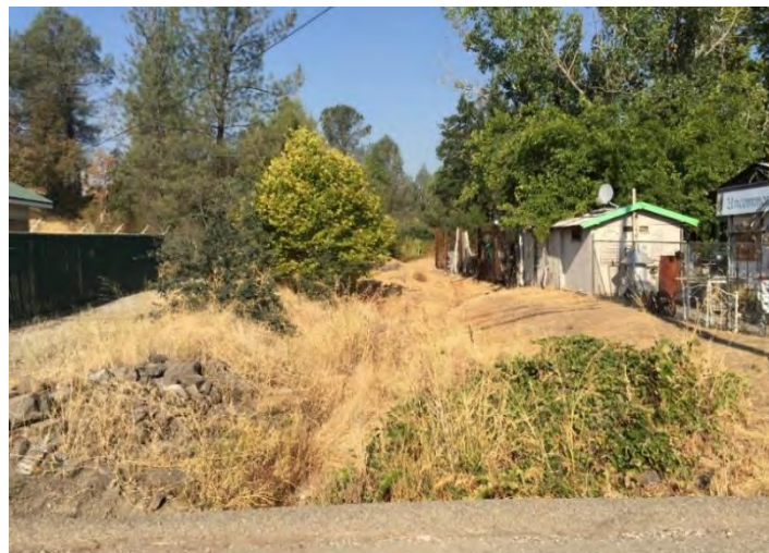
Photo 3.3-2. Cascade Boulevard Drainage Ditch, North of LS3.
