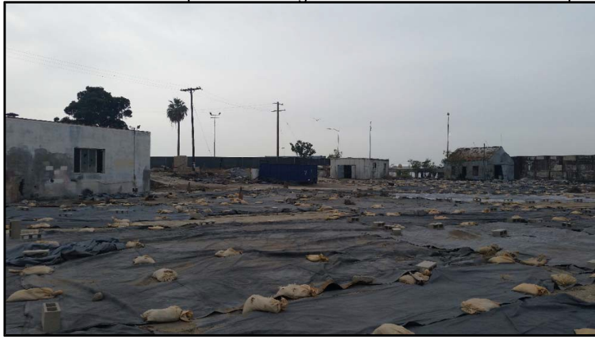
Photo 7. Electrical Shop - the building in the middle with the flat rooftop
