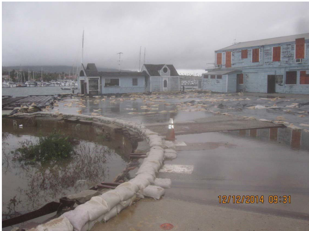
Photo 6 View Looking West with Turntable in the Foreground and Main Building to the Right
