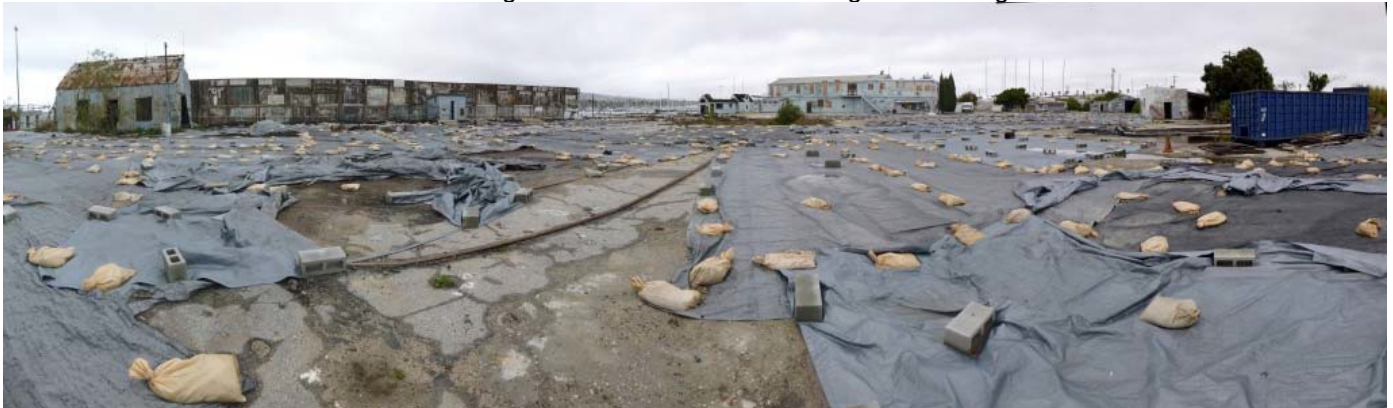
Photo 1: View looking northwest with Main Building in the background
