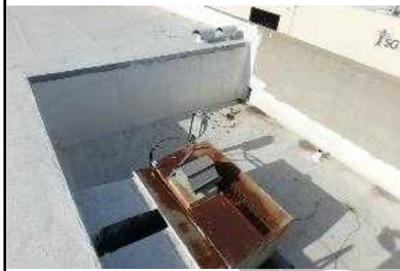
2. Overview of Roof Section 02
