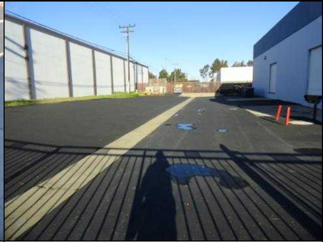
Storm water drainage swales
