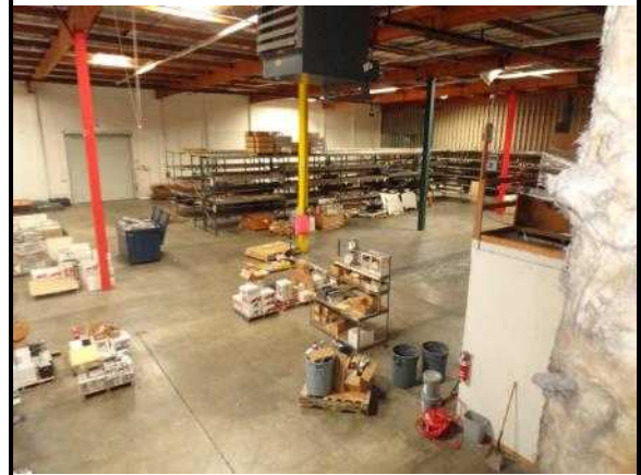
47. Typical warehouse area finishes
