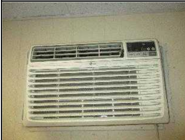
Figure 2.4.3 – Supplemental thru-wall AC
