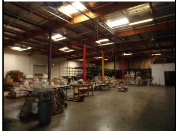
35. Typical roof framing in the warehouse area
