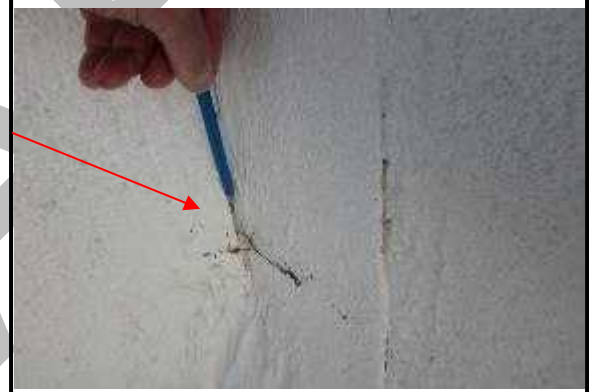
5. Open base flashing seams
