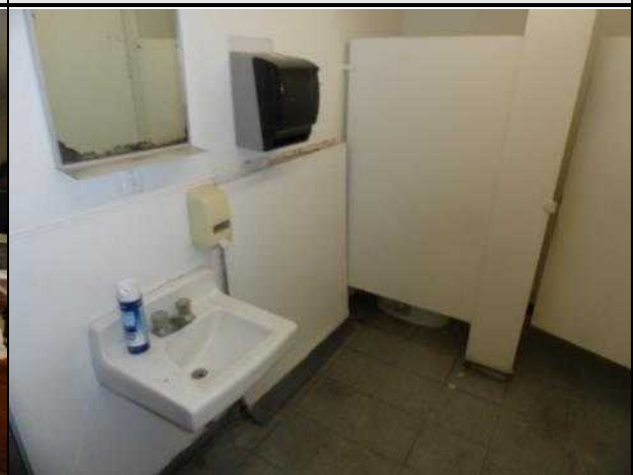
Typical restroom finishes and fixtures
