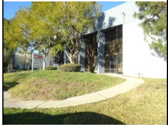
23. Concrete walkway at secondary egress exit from office area
