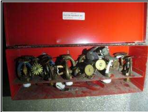
Figure 2.5.3 – Spare sprinkler head box
