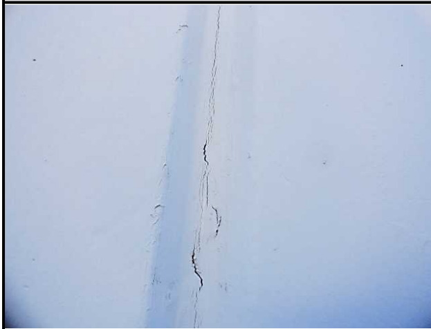
Typical condition of vertical panel joints
