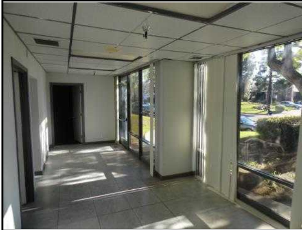
Typical office area finishes on ground floor
