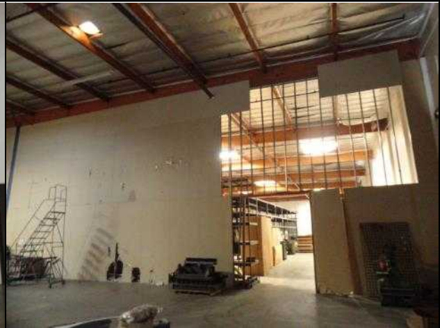
Occupancy separation wall framing between primary tenant space and sub-tenant space
