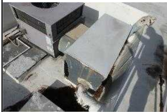
2. Overview of Roof Section 03
