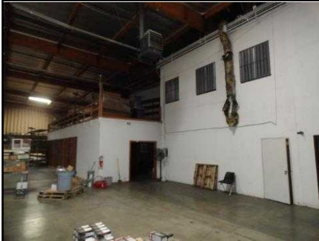
Office area separation walls seen from the warehouse area
