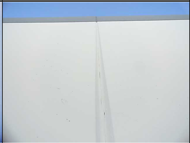
Typical condition of vertical panel joints
