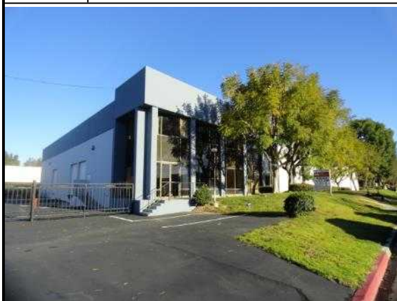
3. Southwest corner elevation showing front south façade and west side facade
