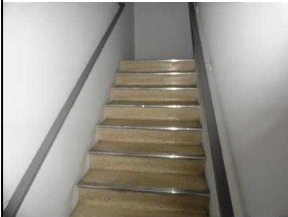
44. Typical stairway finishes
