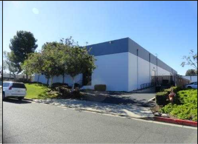
Northeast corner elevation, showing south (front) and east facades
