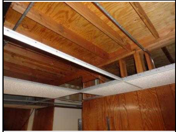
40. Typical framing of second floor deck in office area
