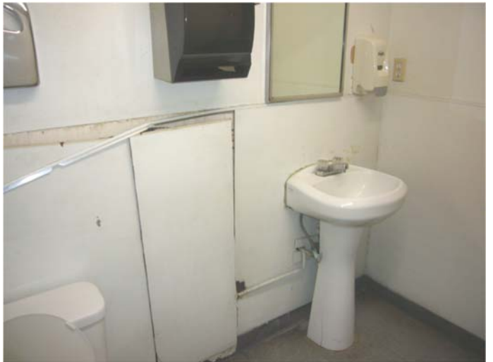
8) View of the typical restroom finishes.
