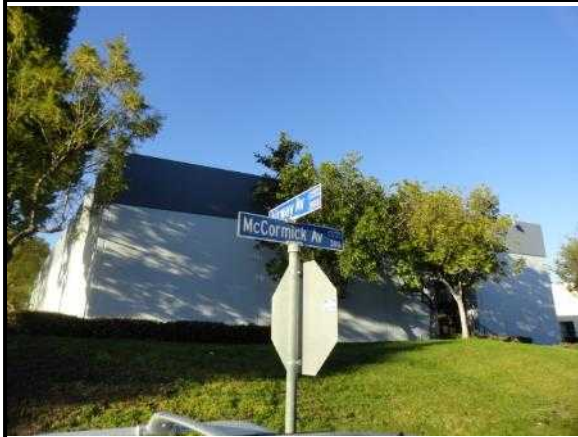
25. Landscaped berms along the east side of the building
