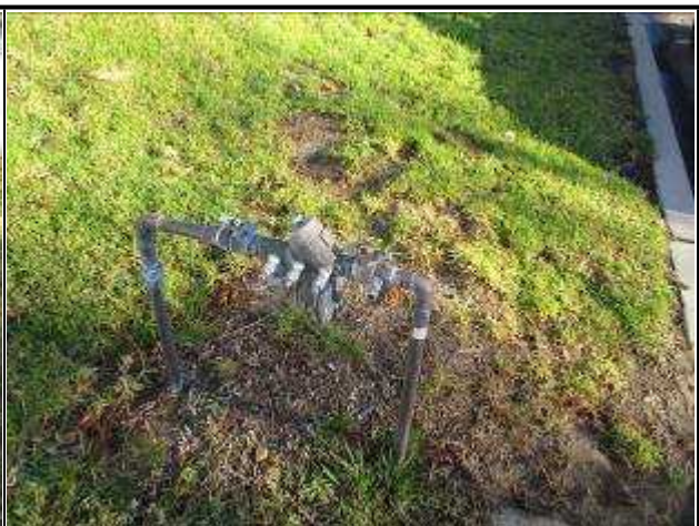
Figure 2.2.2 – Domestic water incoming service
