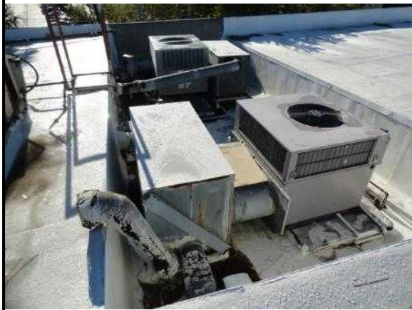
32. Roof in mechanical well over main office area
