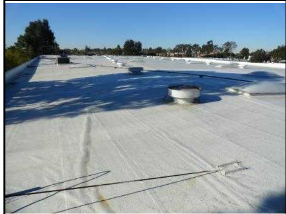
28. Overview of roof
