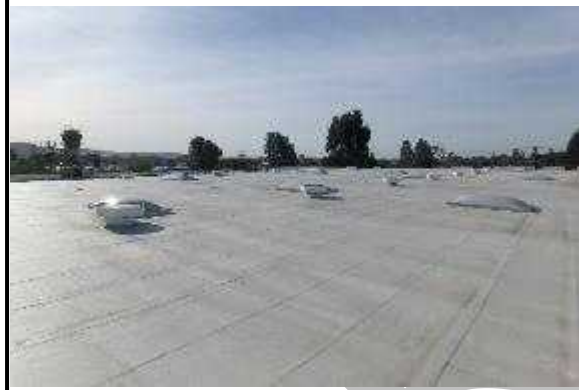
2. Overview of Roof Section 01
