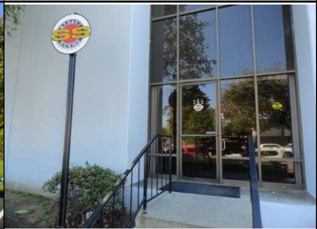
Details at the northeast sub-tenant space entrance
