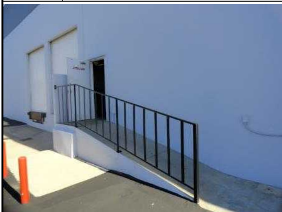
21. Exterior ramp and stairs on west elevation
