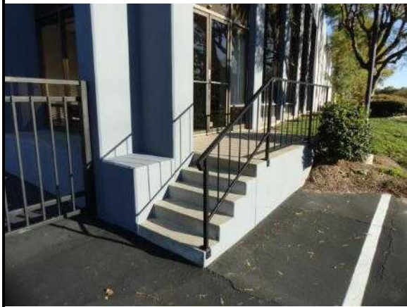
20. Exterior stairs at southwest entrance
