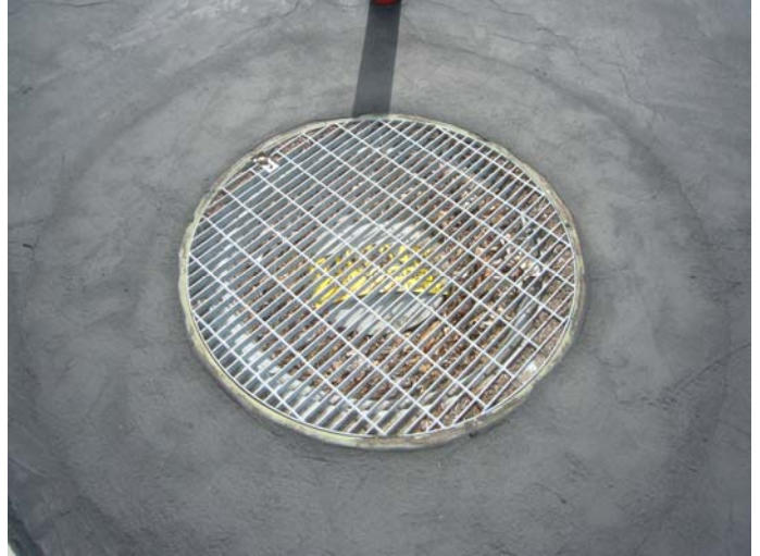
6) View of the electrical transformer vault.
