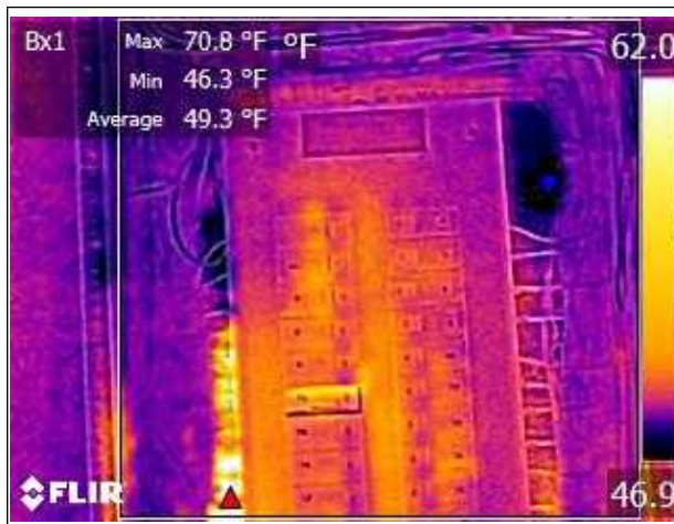
Figure 2.3.7 – Thermal Imaging Sample
