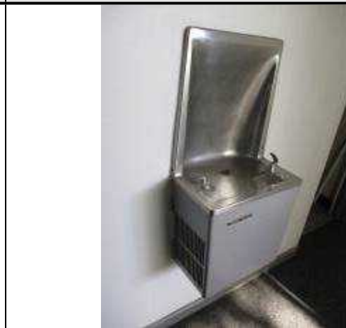
Figure 2.1.6 – Water bubbler
