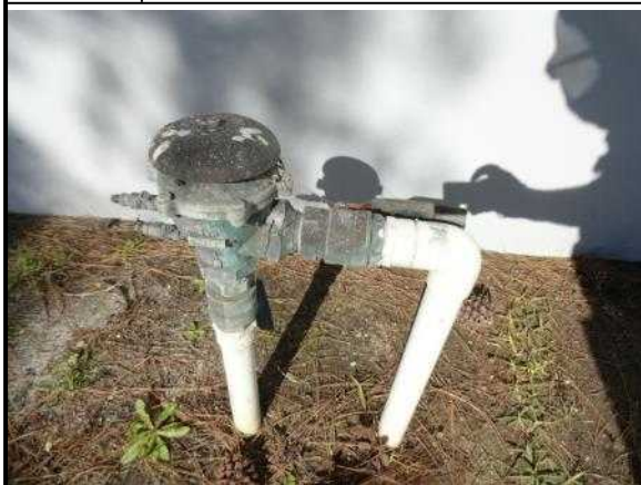
26. Landscape irrigation system backflow preventer
