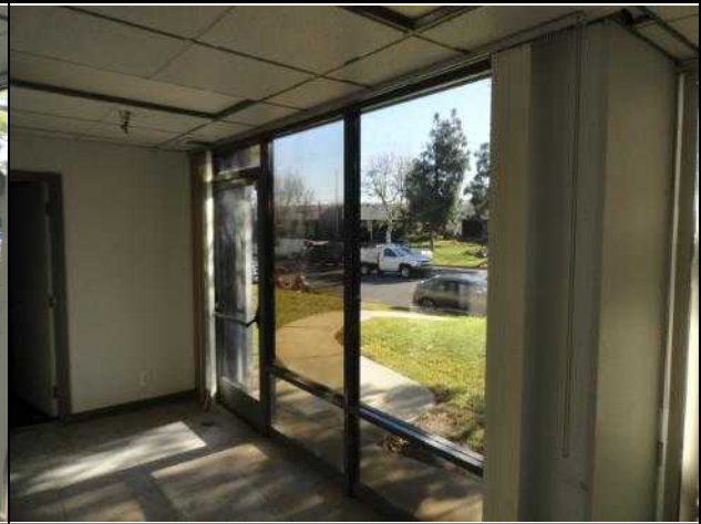
Ground floor office area secondary egress doorway
