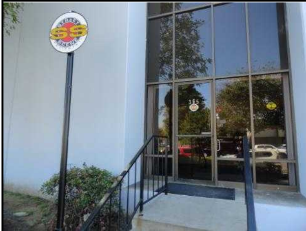
Concrete stairs, railing and signage at the northeast building entrance
