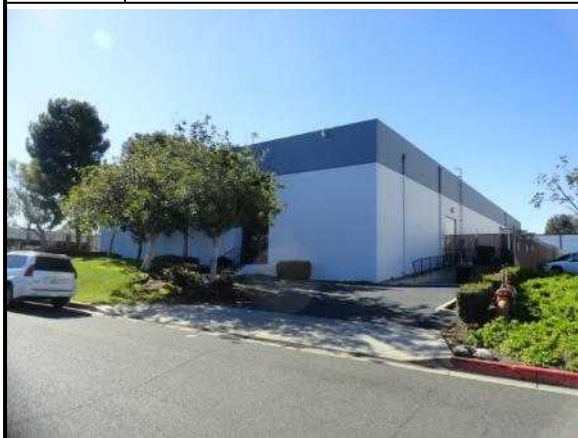
2. Northeast access drive and street view of the property
