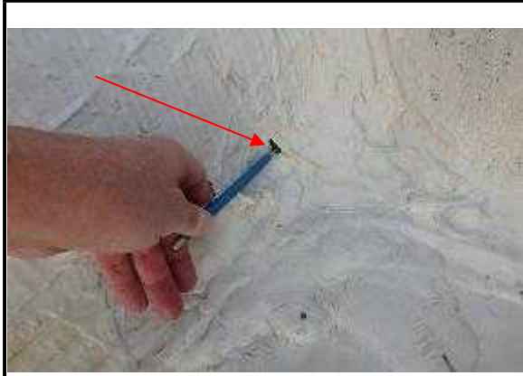
7. Open pin holes on return
