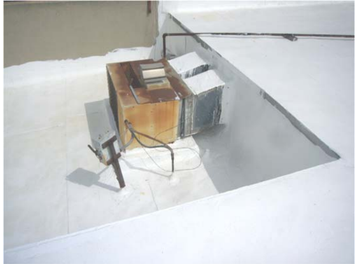
10) View of the roofing and a typical HVAC unit.
