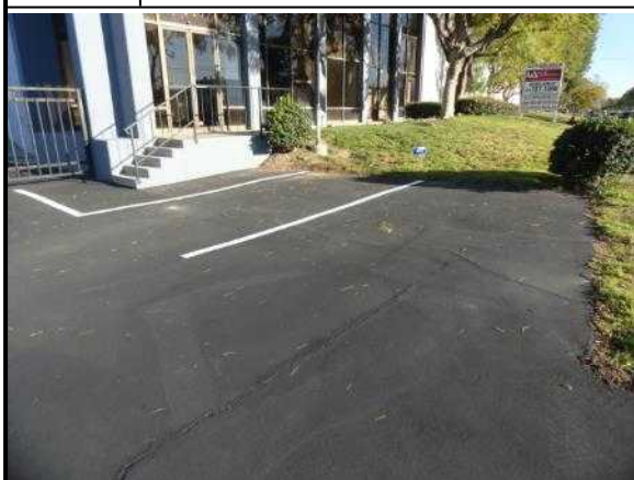
9. Parking spaces at southwest building entrance
