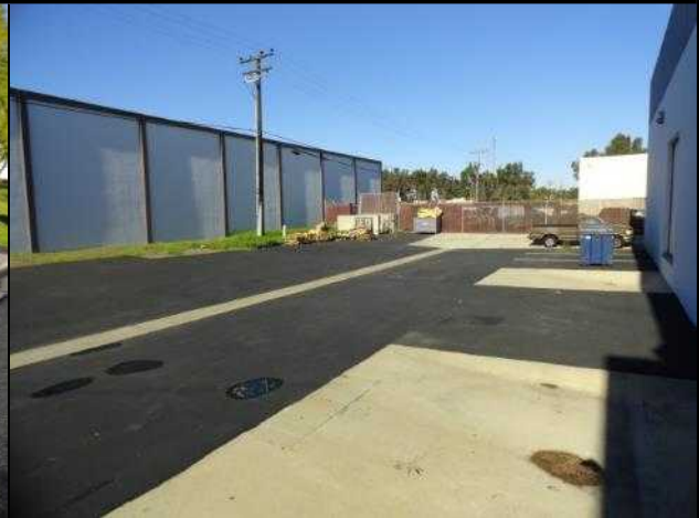
Power is provided from pole-mounted transformers with secondary feeders underground to the main switchboard in the warehouse area
