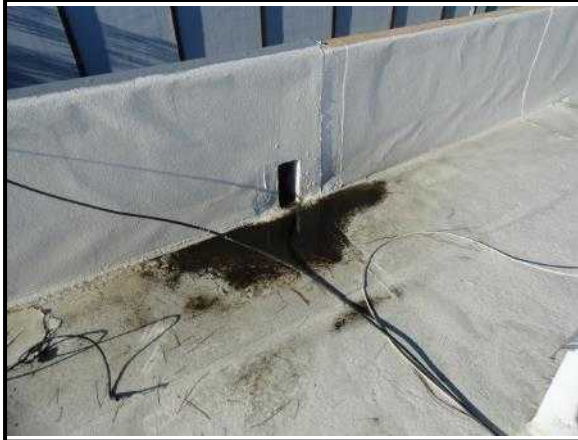
31. Typical parapet drain scupper
