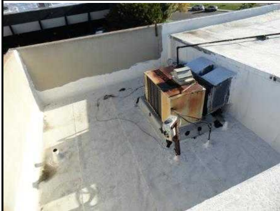
33. Roof in mechanical well over northeast office area
