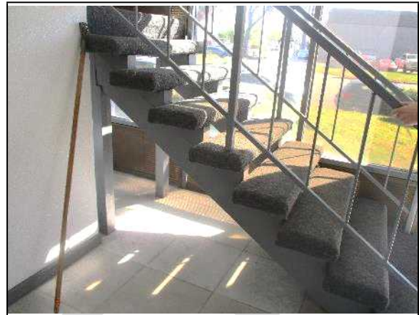
10. Wood framed stairs to office mezzanine.
