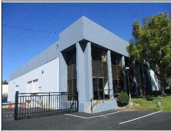
1. View of Subject Property from street. Note storefront system at south east corner.
