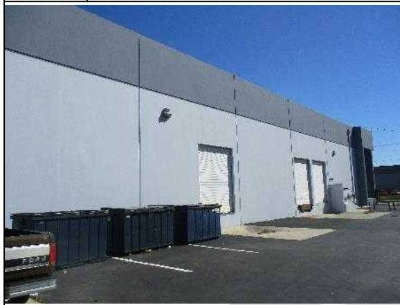
2. Representative façade with some loading dock doors.
