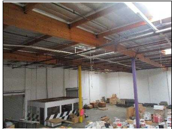
4. Interior of warehouse space.
