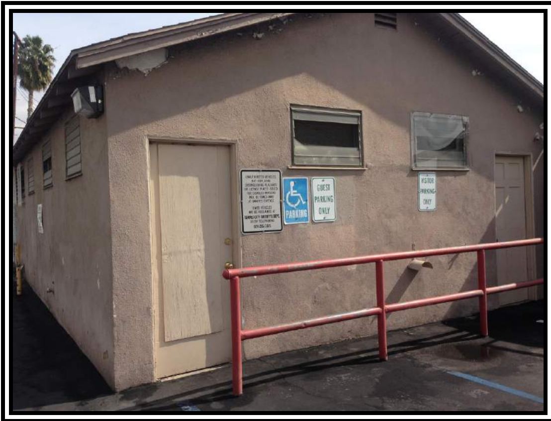
5. 4343 E. LIVE OAK - LAUNDRY ROOM AT NORTH-CENTER AREA OF PARCEL.
