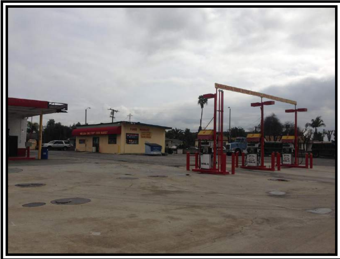
22. ADJACENT - CLOSED CAR WASH/GAS STATION SOUTH OF PROPERTY, SOUTH OF LIVE OAK.
