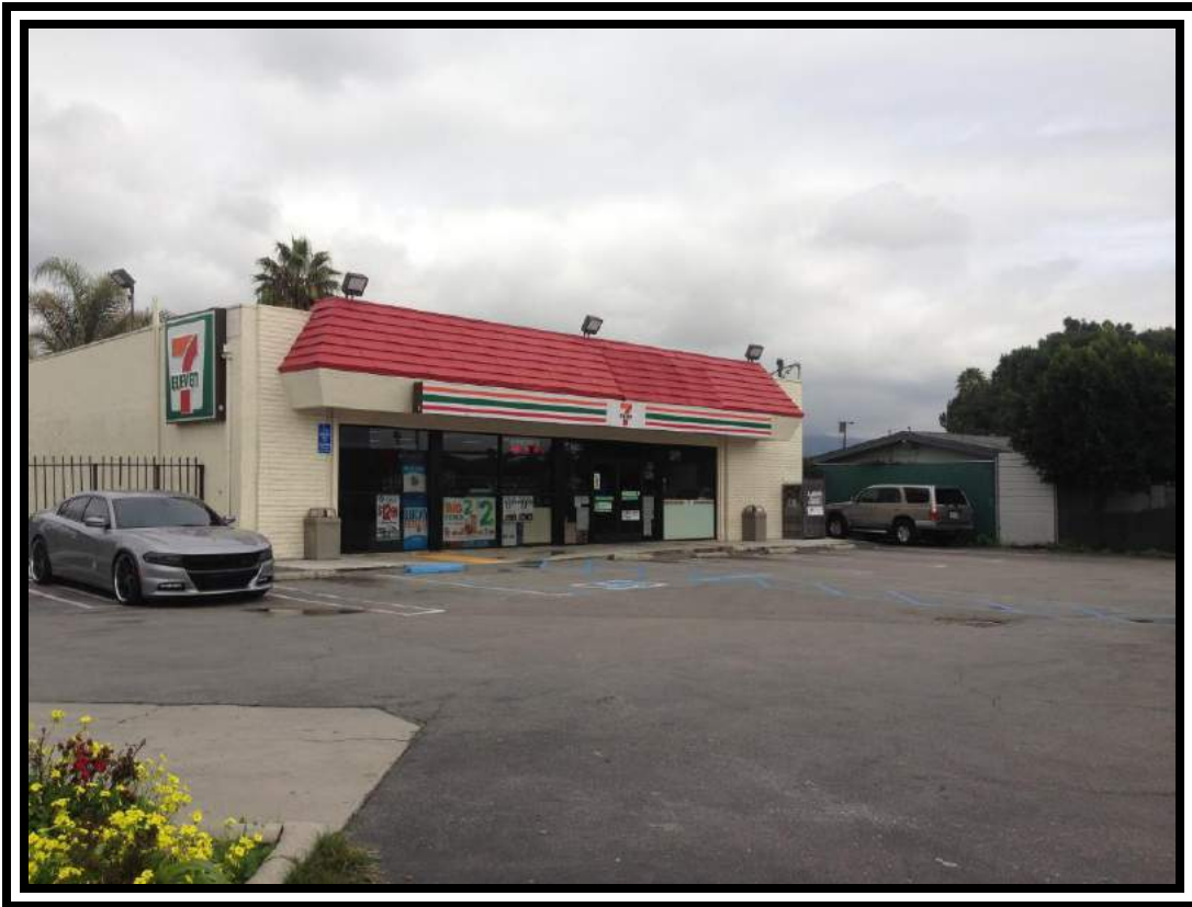
19. ADJACENT - CONVENIENCE STORE ADJOINING SOUTHWEST OF PROPERTY.
