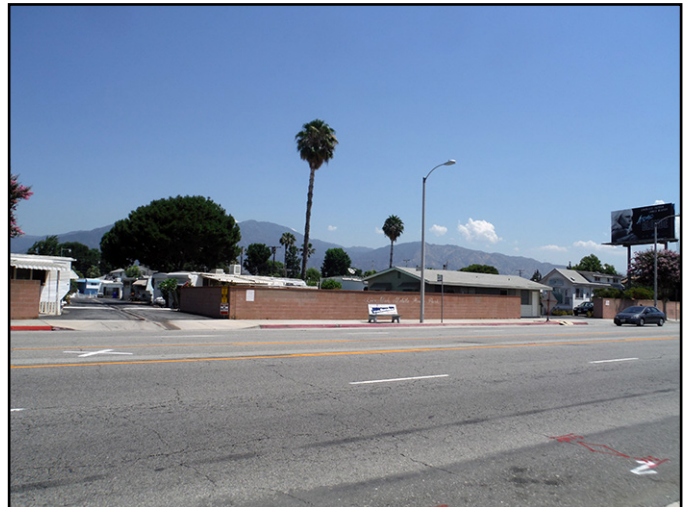
Photo 4 – Northeasterly view of the project site from Live Oak Avenue. Photo taken July 10, 2017.
