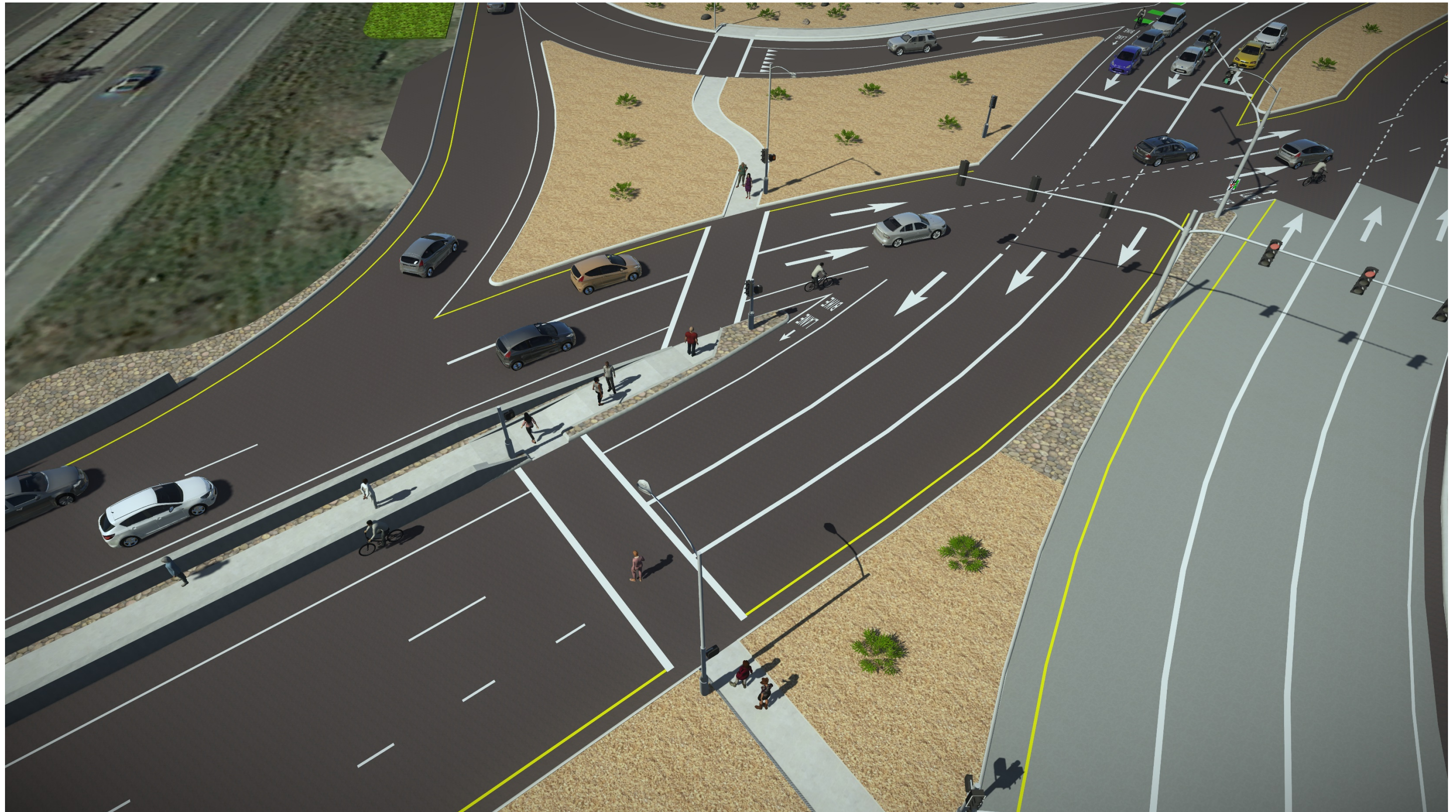
Figure 2-5. North End of Diverging Diamond Interchange Core Looking East *Disclaimer: The Aesthetic features shown in the above simulation are subject to change during the design phase.
