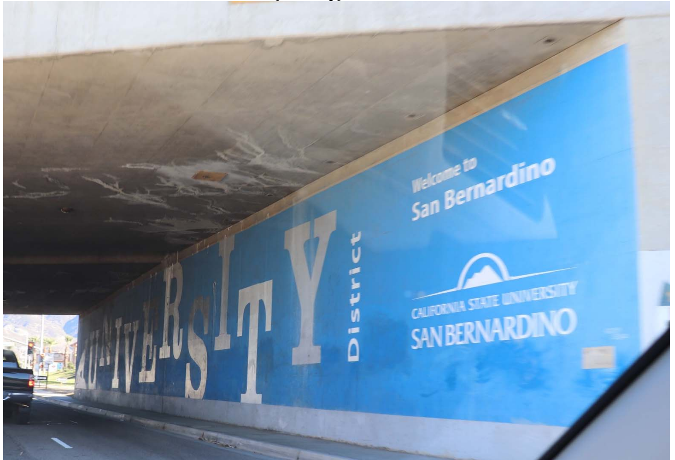
Figure 5. I-215 University Overcrossing Abutment Wall University District Twin Murals – View 2 (Close-Up)
