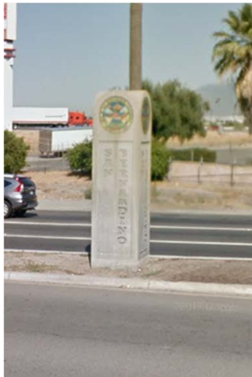
Figure 4. Monument on University Parkway east of I-215/University Parkway Interchange
