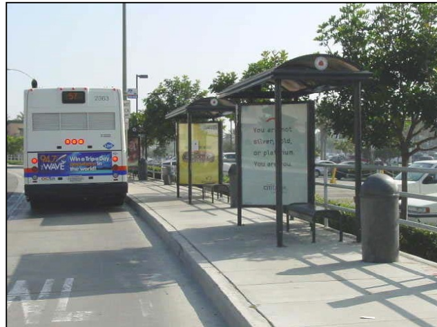
Photo 12: Multiple shelter bus stop.
