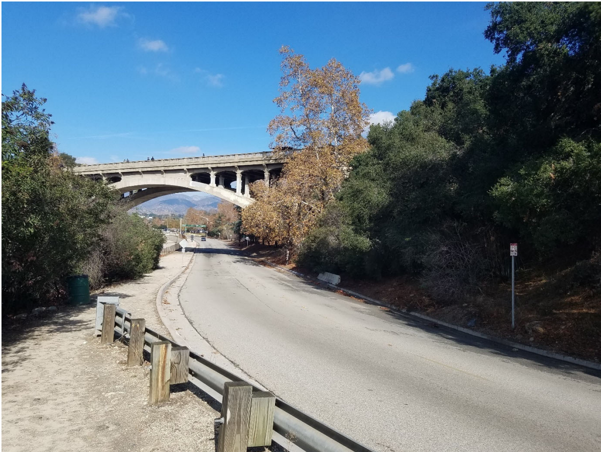
Image showing a view of the existing Holly Street Bridge and North Arroyo Boulevard, looking north towards the bridge.
