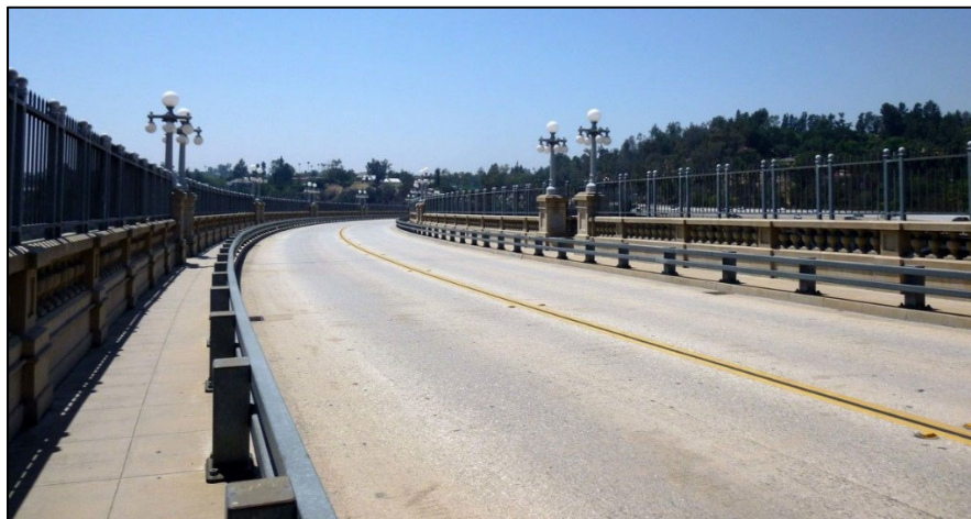
Image showing the existing crash barrier on the Colorado Street Bridge – Similar to what is proposed for the Holly Street Bridge.
