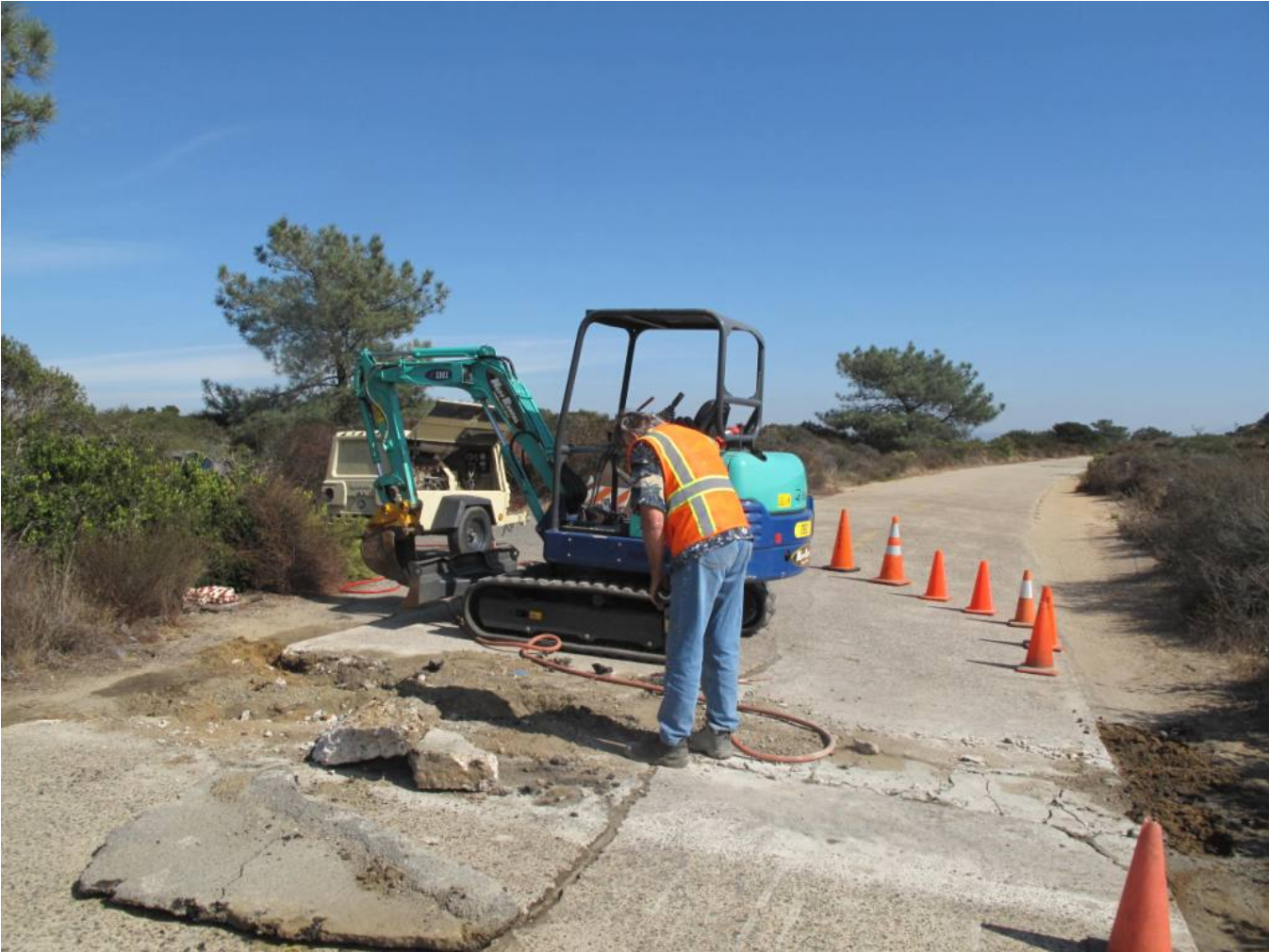
FIGURE 17. TORREY PINES PARK ROAD UNDER REPAIR, NOVEMBER 2011.
