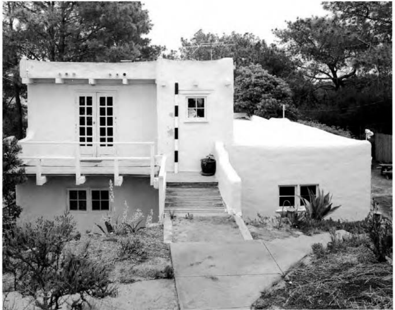
FIGURE 14. GUY AND MARGARET FLEMING HOUSE, VIEW LOOKING EAST. IS ARCHITECTURE, DECEMBER 2006
