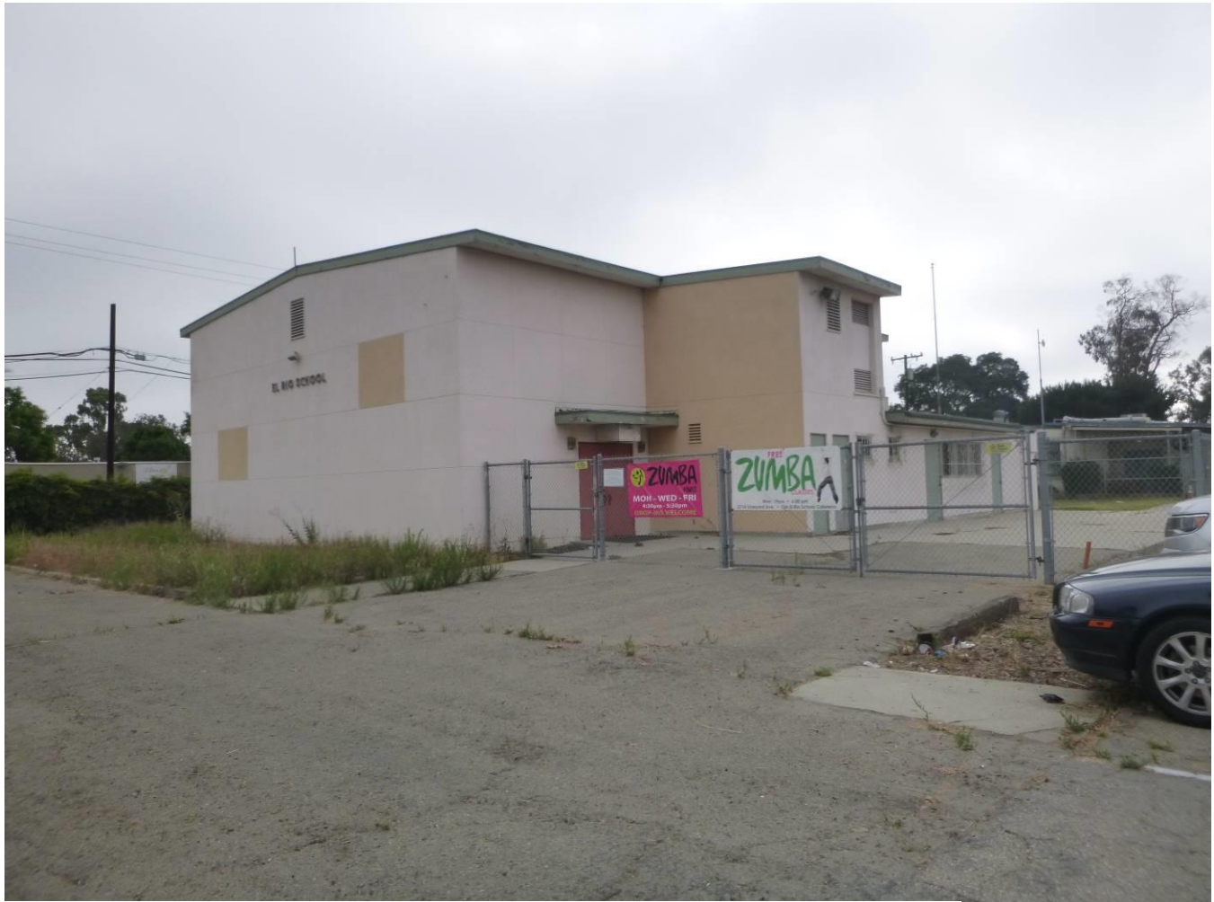
South and west elevations of Building B, facing northeast
