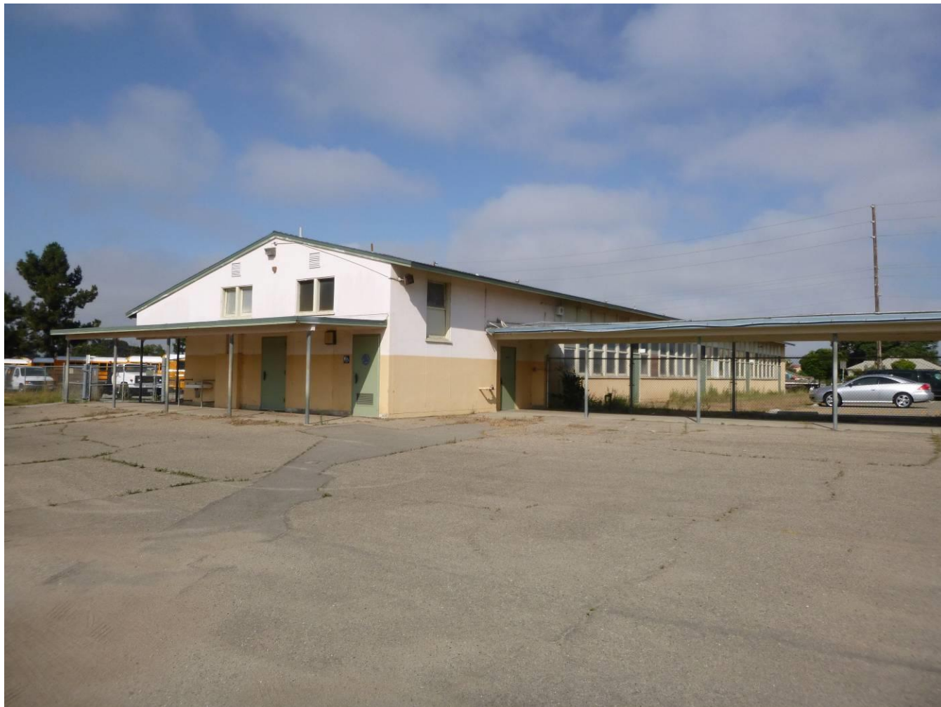
North and east elevations of Building F, facing southwest
