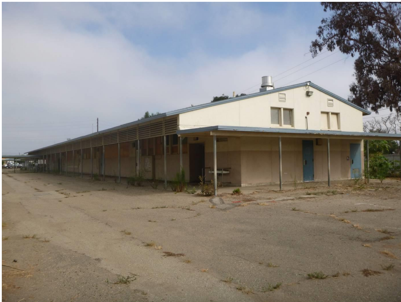
South and east elevations of Building C, facing northwest
