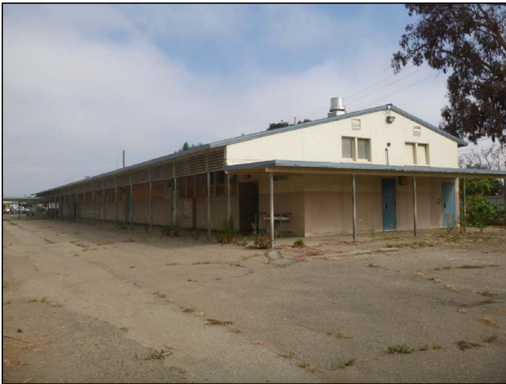
Figure 5-4 South and east elevations of Building C, facing northwest.
