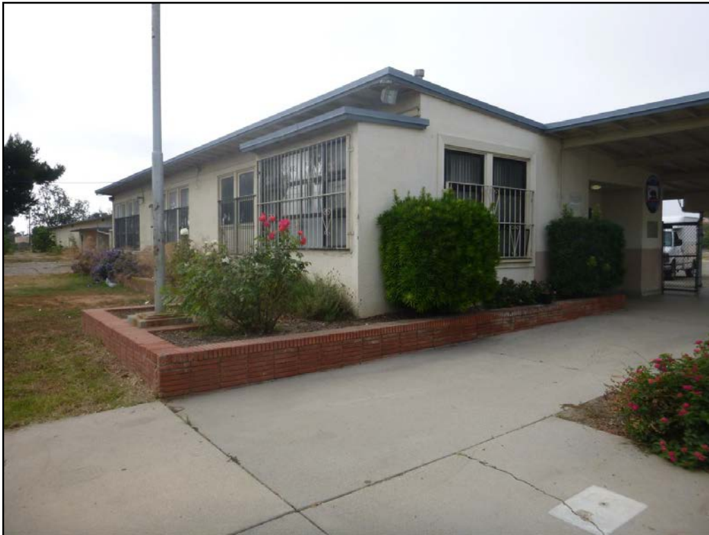
Figure 5-3 North and west elevations of Building A, facing southeast.
