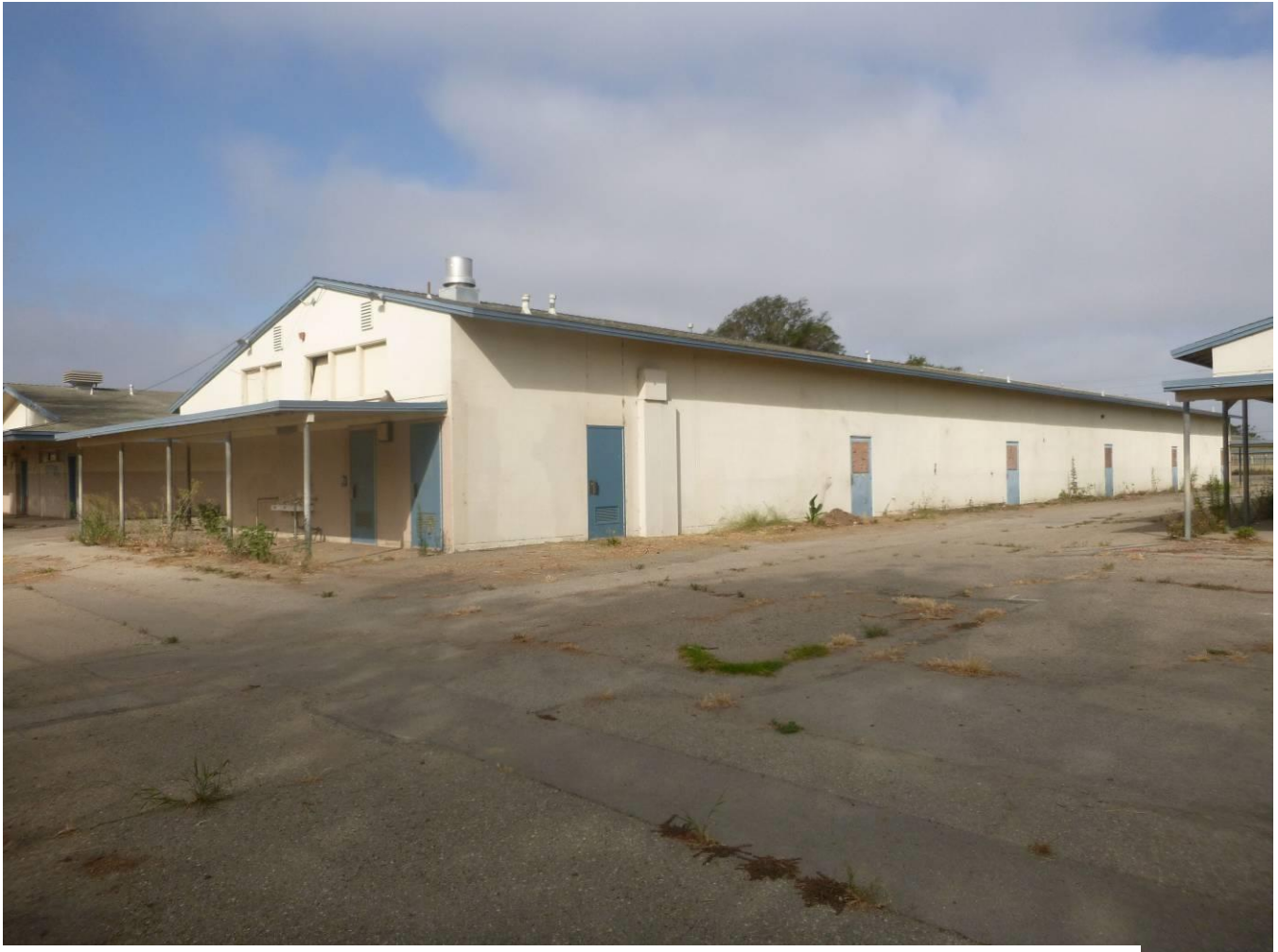
North and east elevations of Building D, facing southwest
