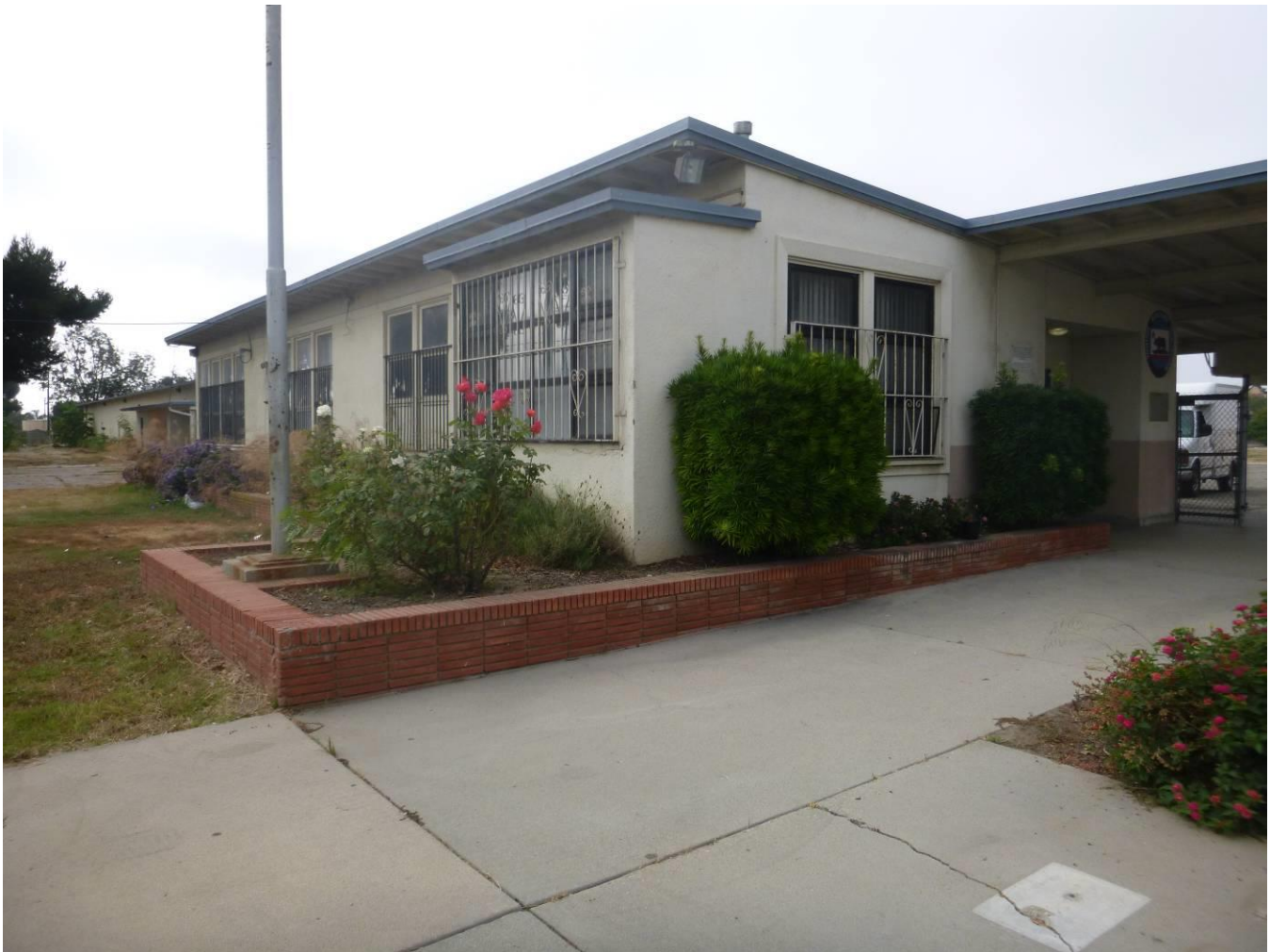
North and west elevations of Building A, facing southeast
