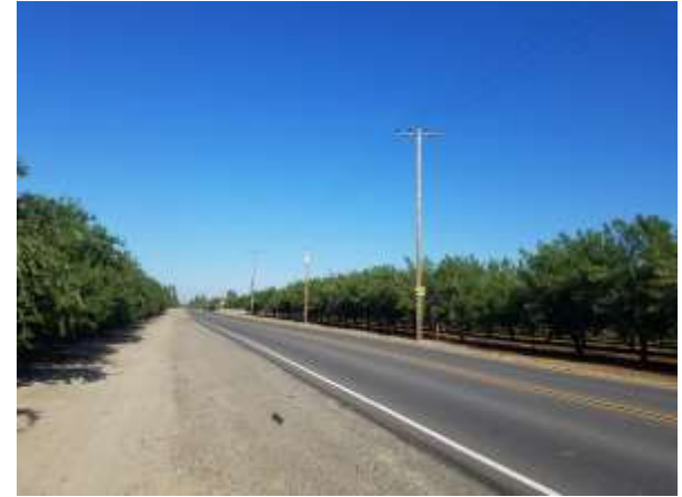
Photograph 9. View of E Keyes Rd east of the canal bridge, looking west.
