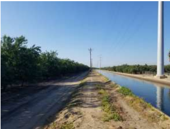
Photograph 10. View of the canal and pole-mounted transformer south of the canal bridge, looking south.
