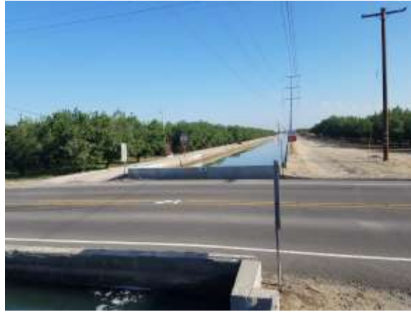
Photograph 2. View of the E Keyes Rd TID canal bridge, facing north.
