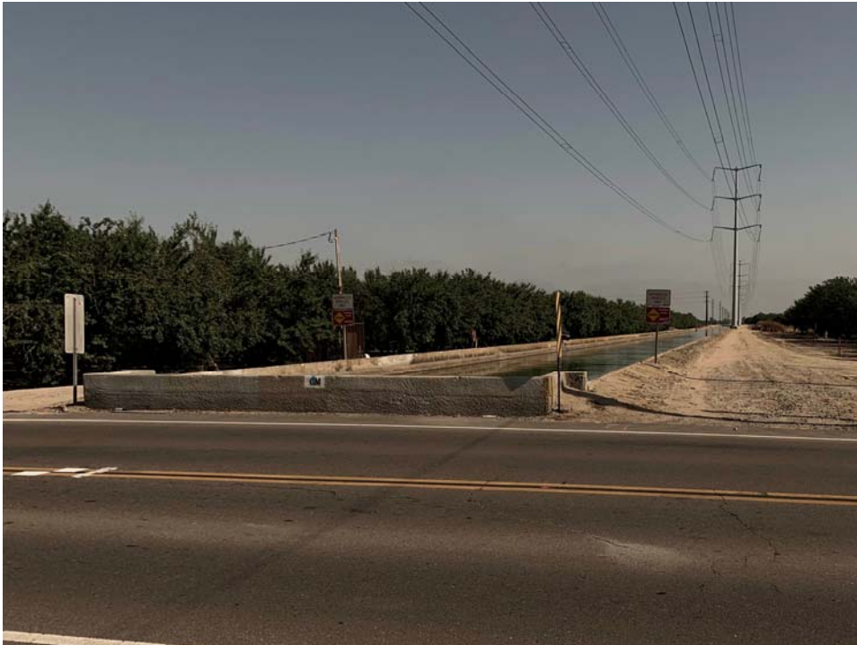
Ceres Main Canal at Keyes Road, camera facing northwest. Photo taken May 9, 2019.
