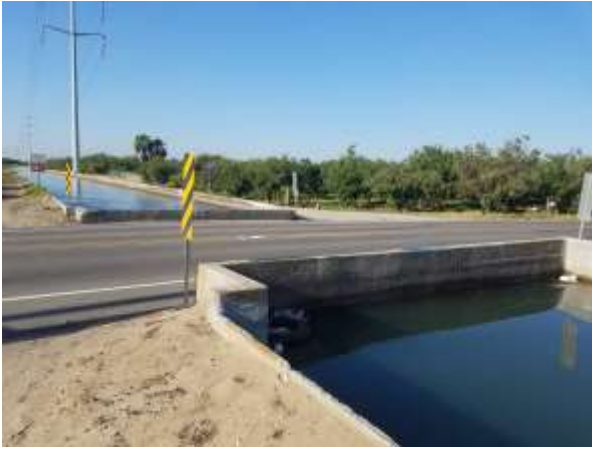
Photograph 1. View of E Keyes Rd TID canal bridge, facing south.
