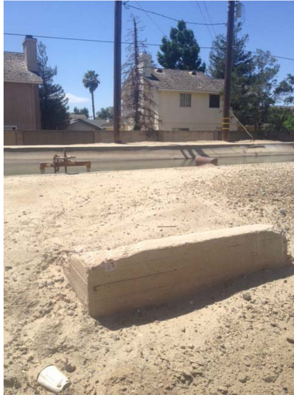
Photo 753. Feature A - cement foundation and pipe (right background) on the east side of the canal in the berm, adjacent to an intake valve (left background). Facing west.
