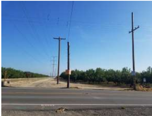
Photograph 5. View of northeastern corner of canal bridge where three utility poles are located, looking north.
