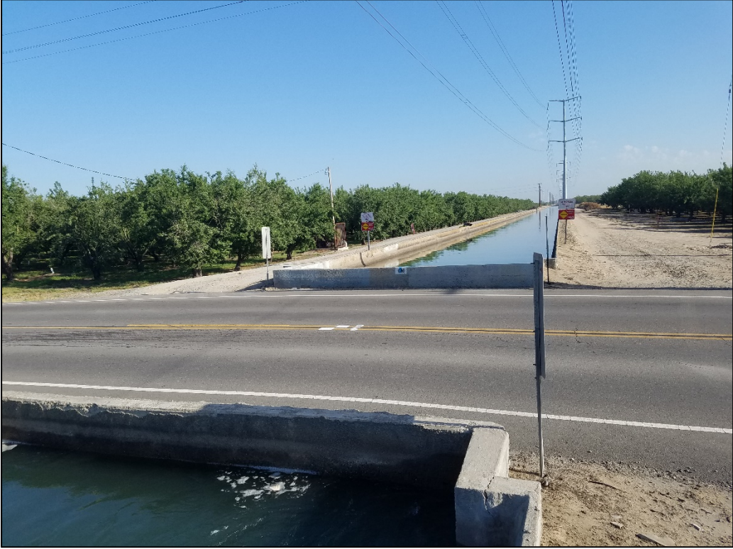
Figure 4 Transmission Lines along TID Canal, Bridge in Foreground
