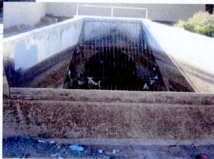
No. 2. Lateral 1 at Ceres Main Canal, view west.
