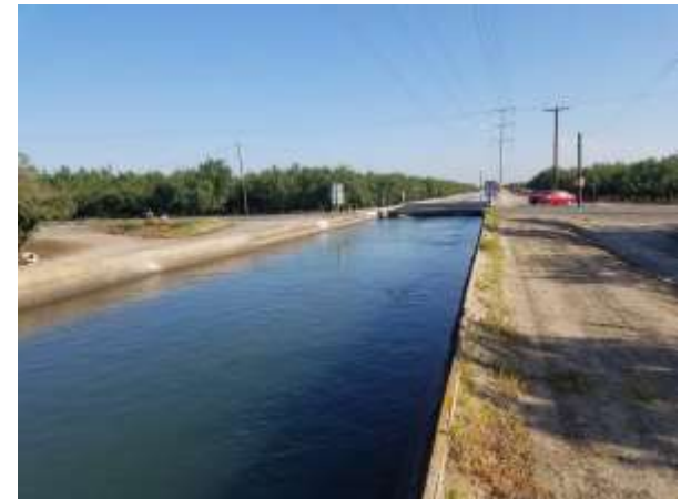
Photograph 12. View of canal bridge from southern project site boundary, looking north.
