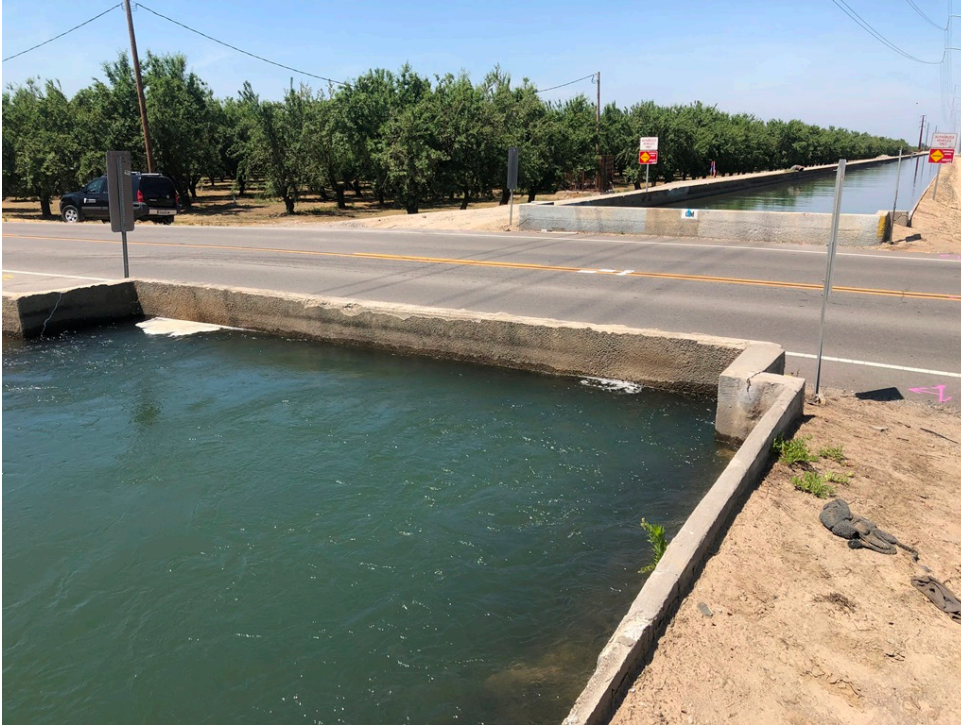
Photograph 1. Ceres Main Canal under Keyes Road. View to the north west.
