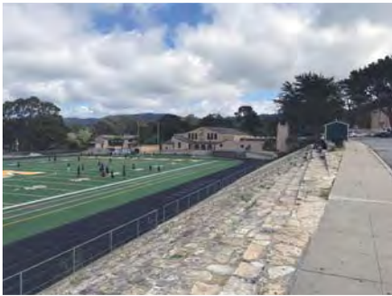
② View from top of existing stadium seating (looking south)
