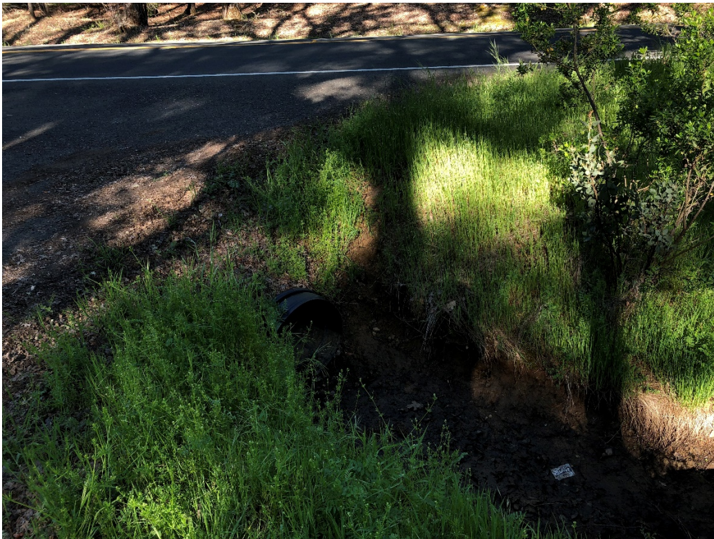
Photo 6 – Class III road crossing (east side)
