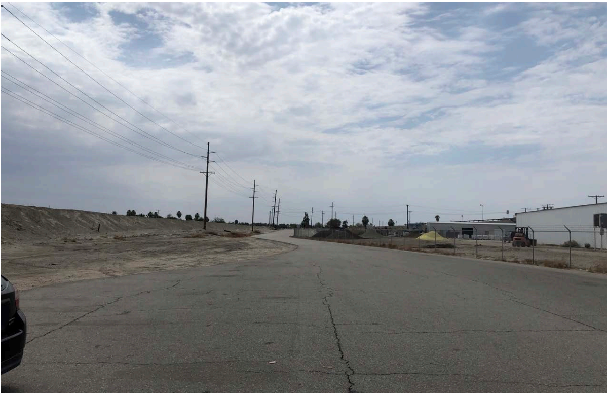
Photograph 4. South facing view of paved roads and development within the APE.
