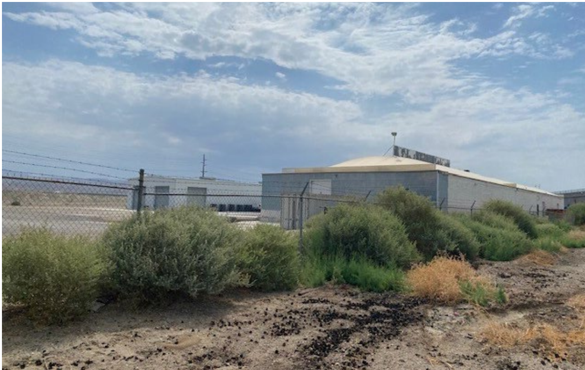
Photograph 5 87400 Airport Blvd., Facing Southeast
