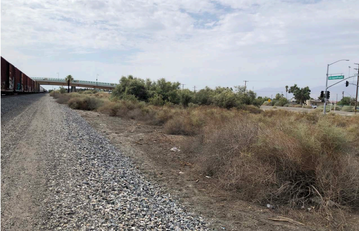
Photograph 3. South facing photo of quailbush scrub habitat along the railroad tracks within the APE.
