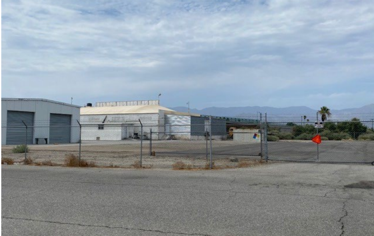
Photograph 4 87400 Airport Blvd., Facing East
