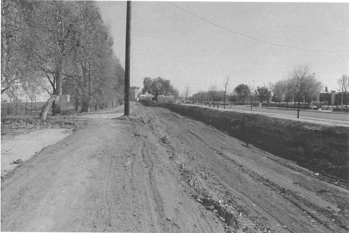
FIGURE 7 : VIEW LOOKING EAST NEAR PROPOSED BRIDGE LOCATION. (PHOTO TAKEN MARCH 9, 2018)
