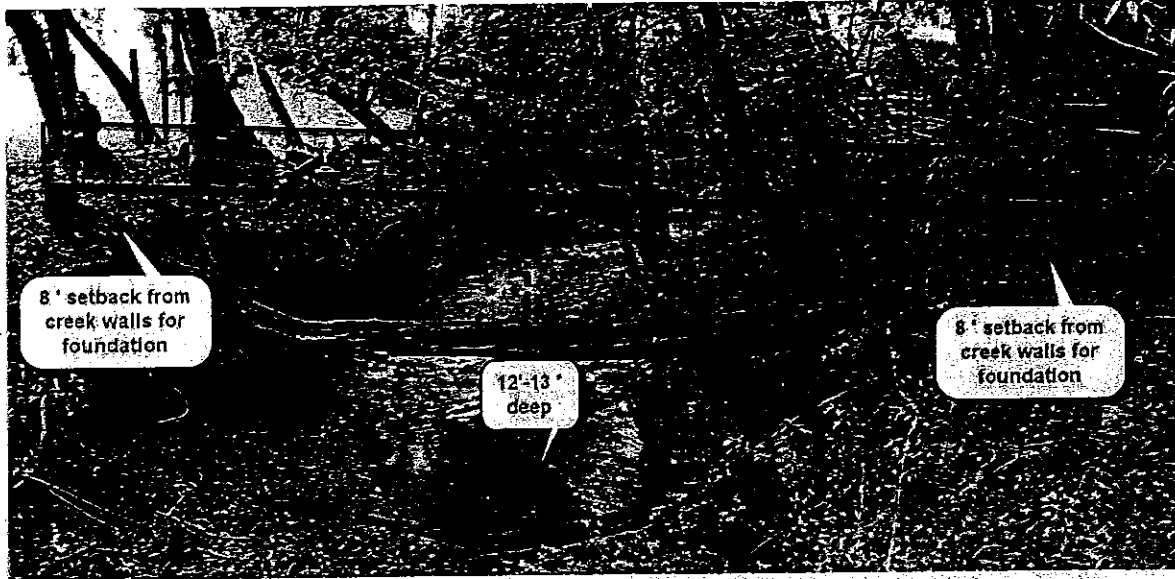
Detail pictures of the footing/abutment setbacks
