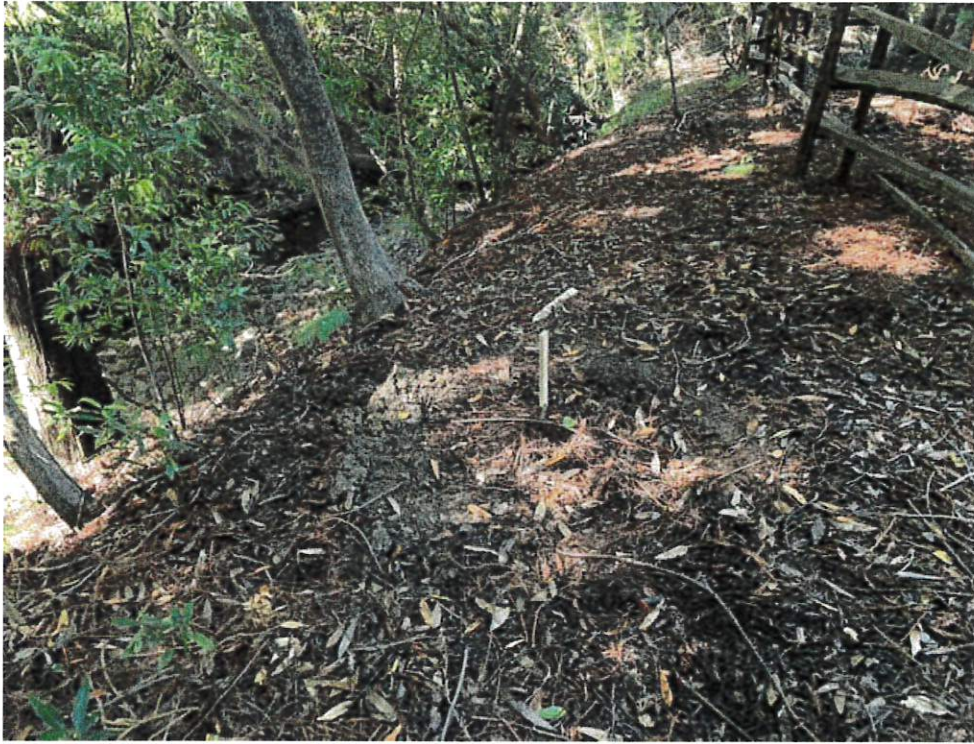
Appendix B-7. Location of proposed bridge footing, above north top-of-bank of Bear Gulch Creek, looking downstream.
