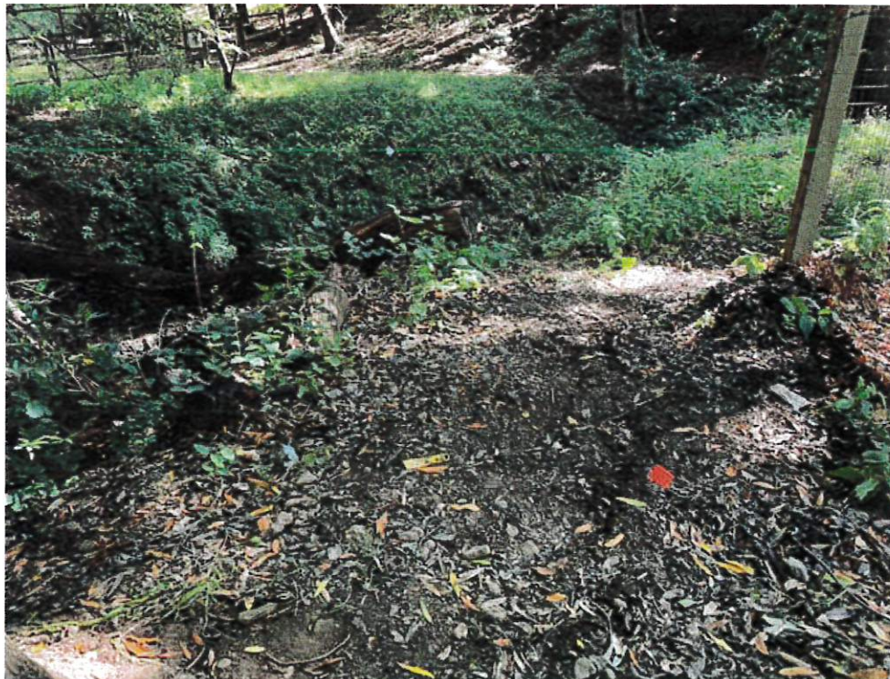
Appendix B-6. Location of proposed bridge footing, above south top-of-bank of Bear Gulch Creek, looking upstream.
