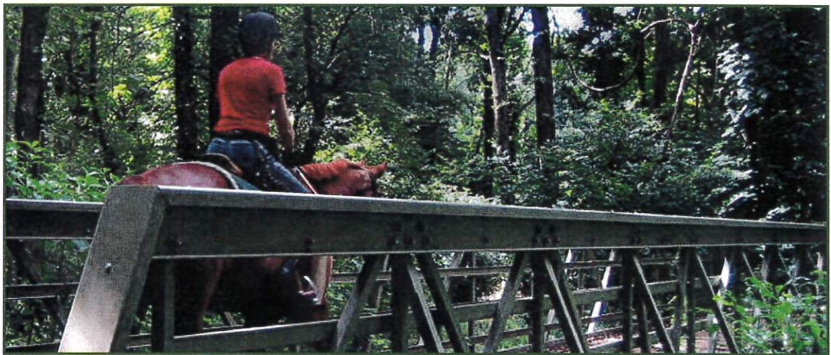
Figure 10. Prototype of the proposed Fiberglass Reinforced Polymer (FRP) bridge.
