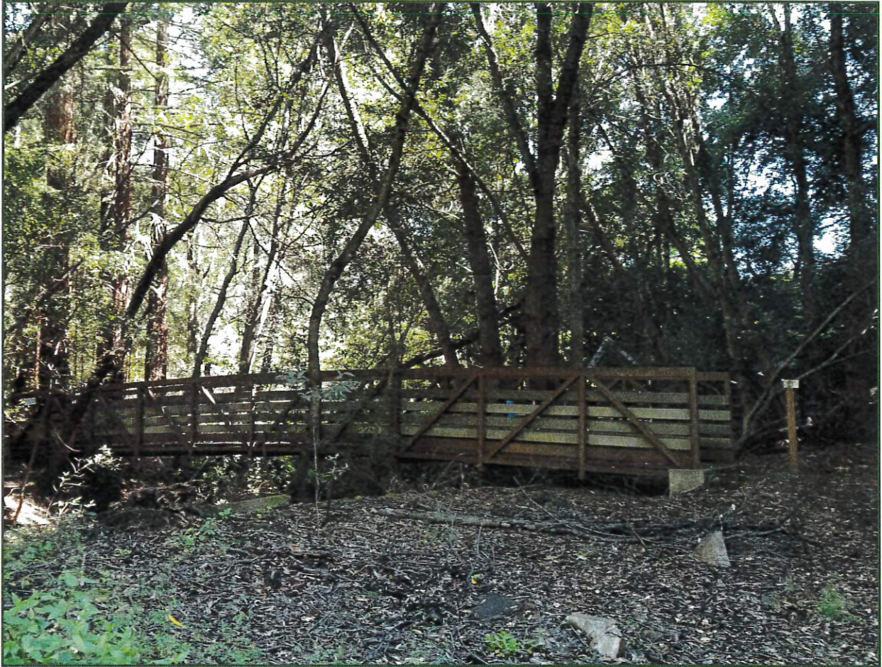
Figure 5. The “Old Metal Bridge” upstream of the project site, constructed approximately 20 years ago after an initial washout of the Center Trail.
