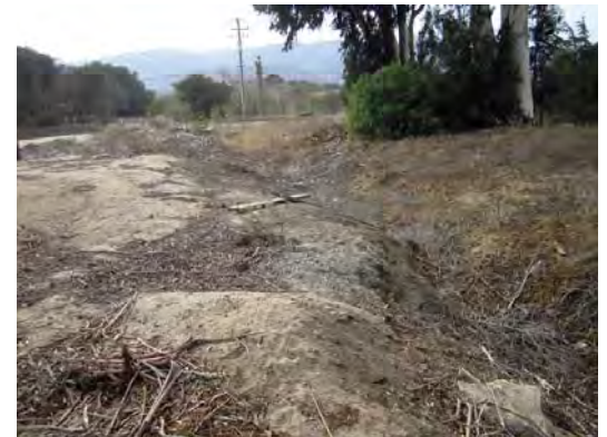
④ Drainage channel, looking southwest
