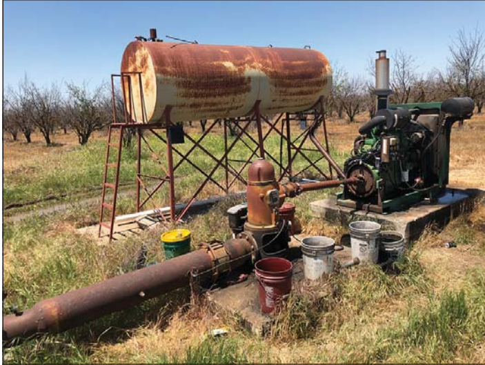
PHOTOGRAPH 8: View of Diesel AST, diesel engine, and nine empty buckets
