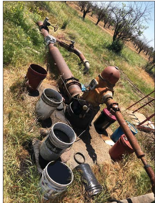
PHOTOGRAPH 11: Eight out of nine observed buckets
