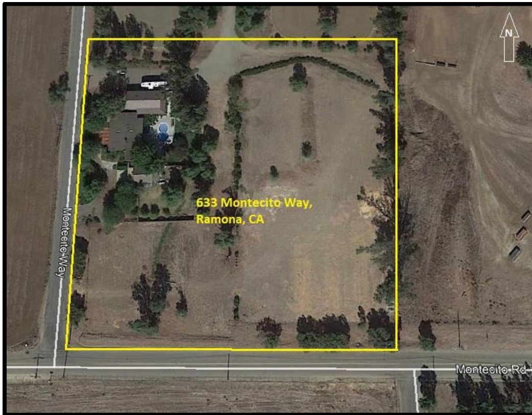
Photo 1. View of Existing Project Site on Montecito Way.
