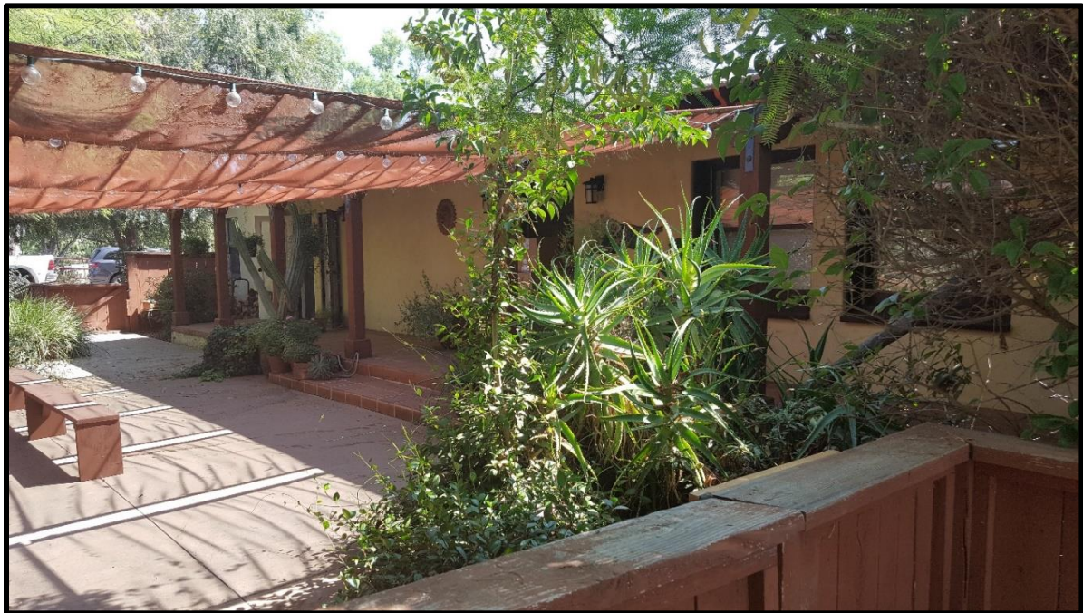
Photo 4. View of the front of the Ranch House.
