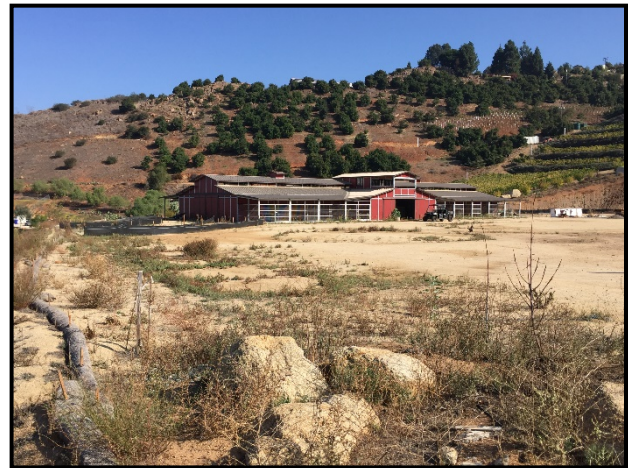
Photograph 4. Photo of south side of building, facing north. Graded area is proposed for corral and open stables. Avocado orchard, vineyards are on hillside behind horse stable.
