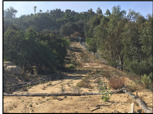
Photograph 6. photograph of proposed driveway (graded area), which connects to Highland Valley Road.
