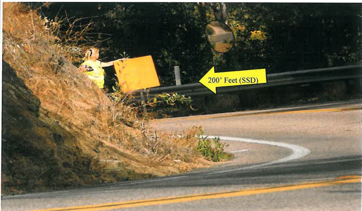
Looking West on Highland Valley Road to provide 200' Feet of Stopping Sight Distance (SSD) from the projects driveway. (Zoomed In)
