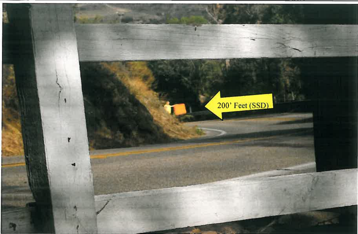
Looking West on Highland Valley Road to provide 200' Feet of Stopping Sight Distance (SSD) from the projects driveway.
