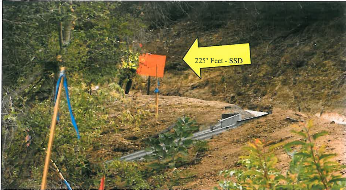
Looking East on Highland Valley Road from the projects driveway to provide 225' Feet Stopping Sight Distance (SSD).
