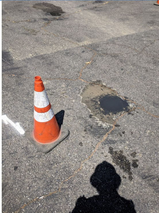
PHOTO 5: Patched asphalt following completion of drilling (7/16/19).
