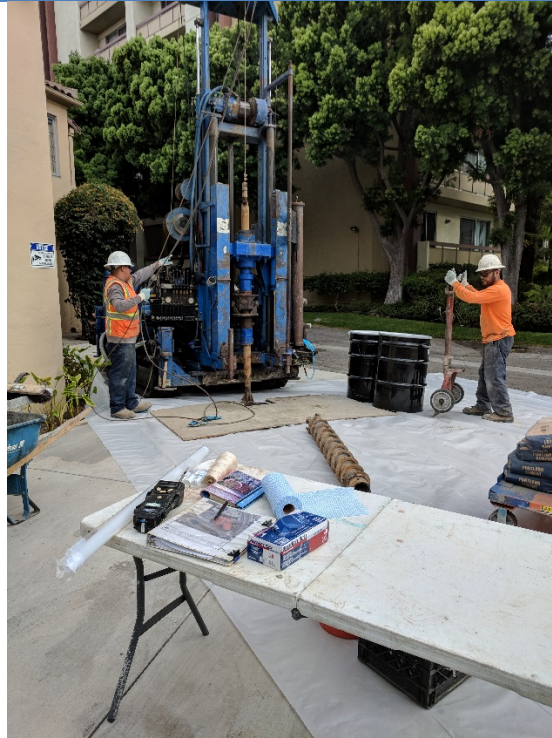
PHOTO 9: Drilling at location B5 with the limited access rig (7/18/19).
