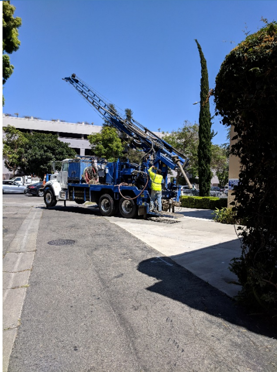
PHOTO 7: Setting up at boring B5 (7/17/19)
