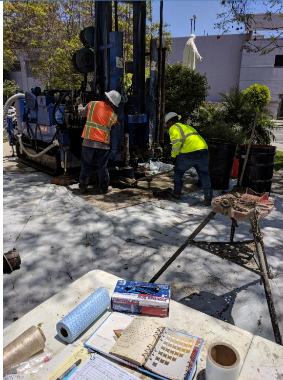
PHOTO 11: Drilling in the grass at location B6 with the limited access rig (7/18/19).
