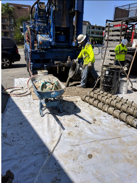
PHOTO 4: Backfilling with bentonite grout (B1) (7/16/19).
