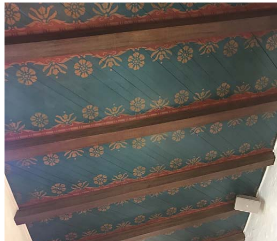
Cathedral interior, view of original stenciled/painted ceiling at side aisle (ARG, 2018)
