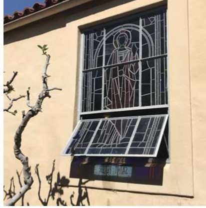
Cathedral, view of typical non-original stained glass/ steel window (ARG, 2018)
