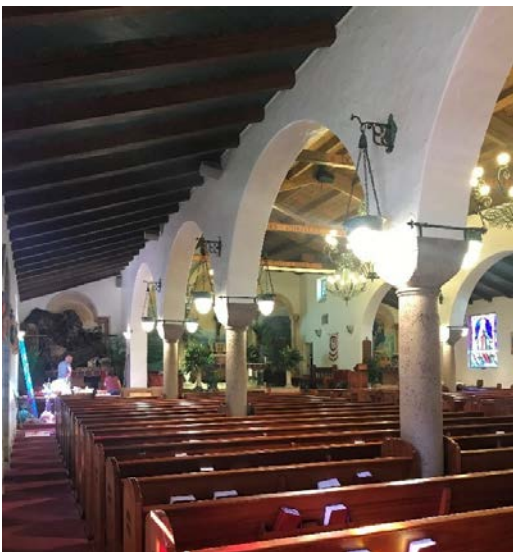
Cathedral interior, west side aisle, view northwest (ARG, 2018)
