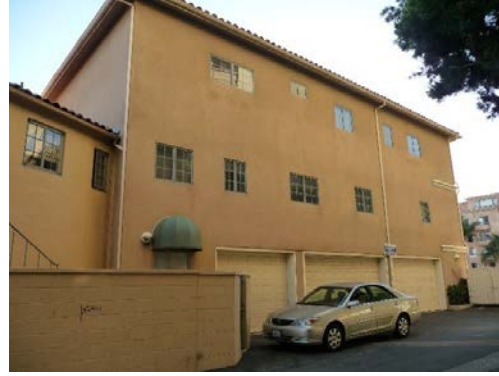
Chancery, view southwest (ARG, 2016)
