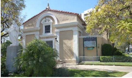
Front façade of the cathedral, 2016. Note the replaced window above the primary door and the added rounded bay to the right of the primary entrance volume, compared to the historic image at right.
