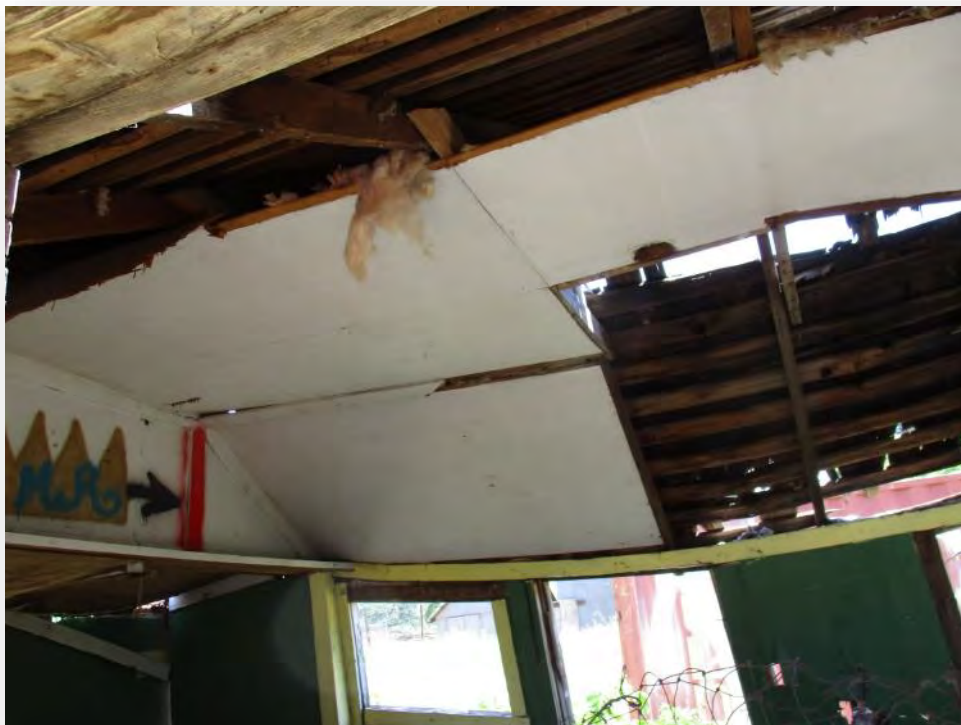
Photo 18 – Interior of small shed.
