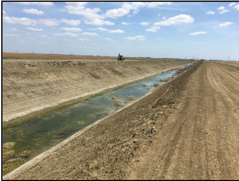
Canal along Laurel Avenue facing east
