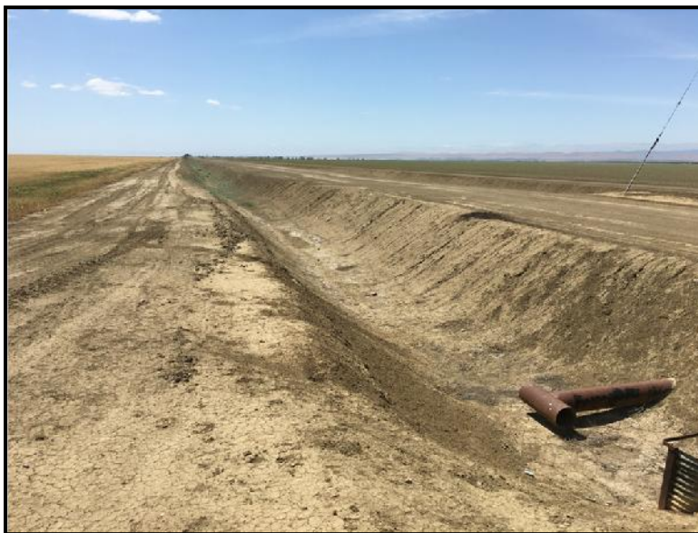
Unpaved canal at west boundary of Site facing south
