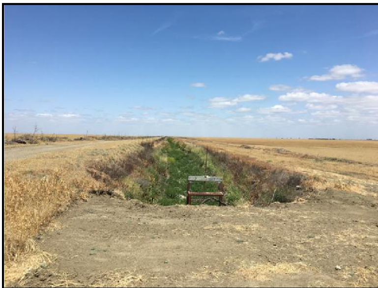
Unpaved canal in east portion of Site facing north
