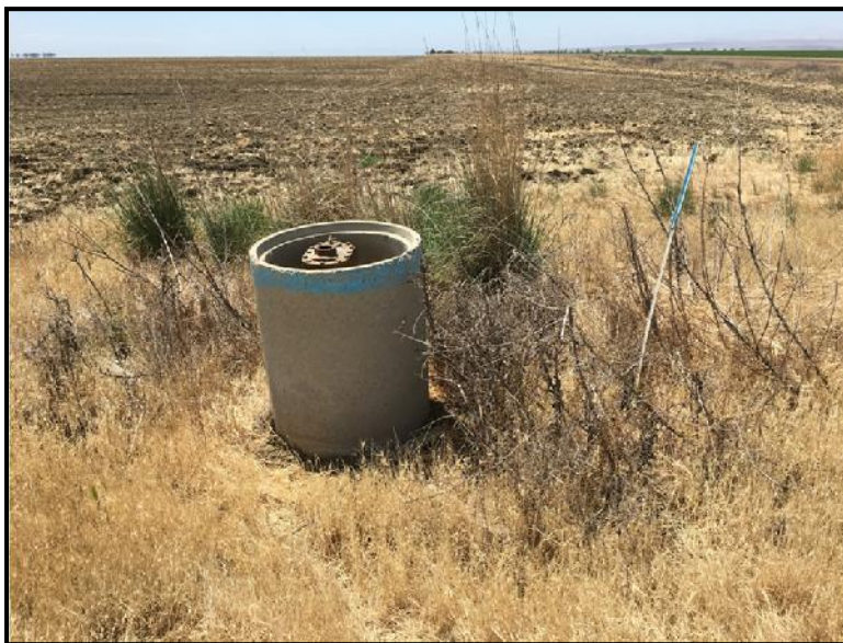
Example of concrete standpipe with pump located throughout Site
