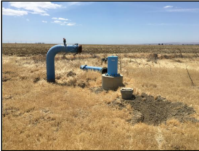
Example of agricultural pipes throughout Site
