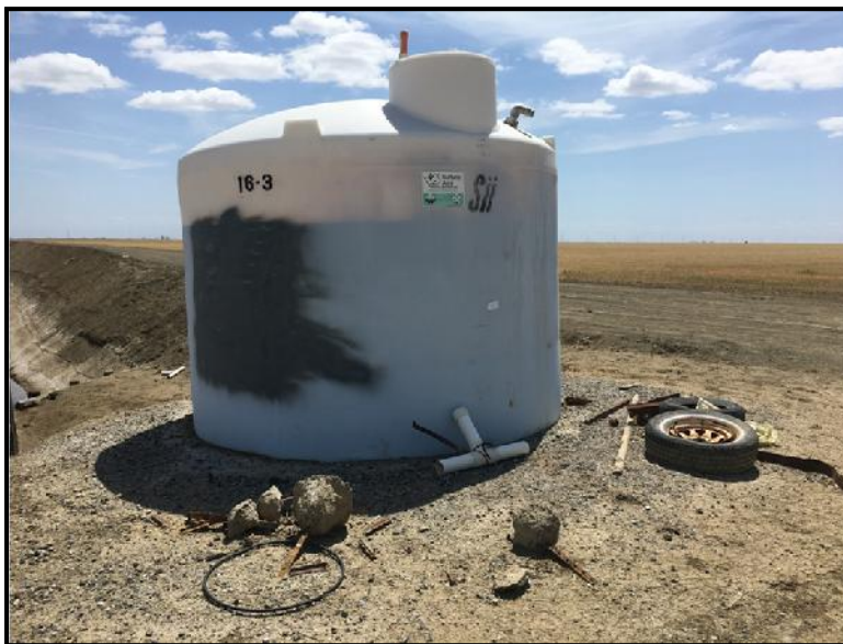
4,000-gallon poly tank containing Sulfuric Acid in northwest corner of Site
