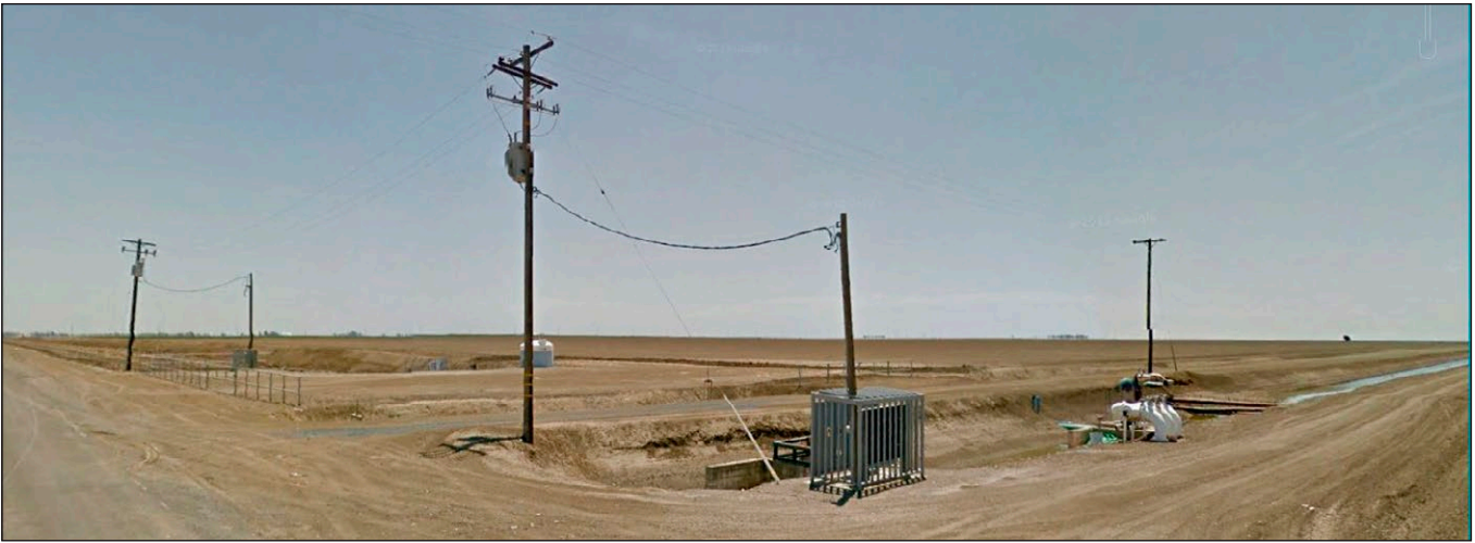
Photo 1: Southeastward view from northwest corner of site.
