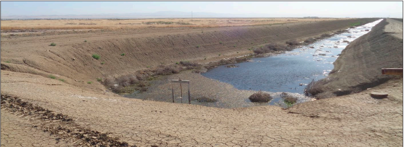
Photo 2: Westward view toward site from south side of Laurel Ave. at 25th Ave.
