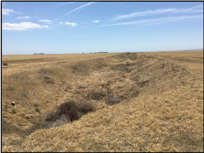
Unlined canal on Site facing south
