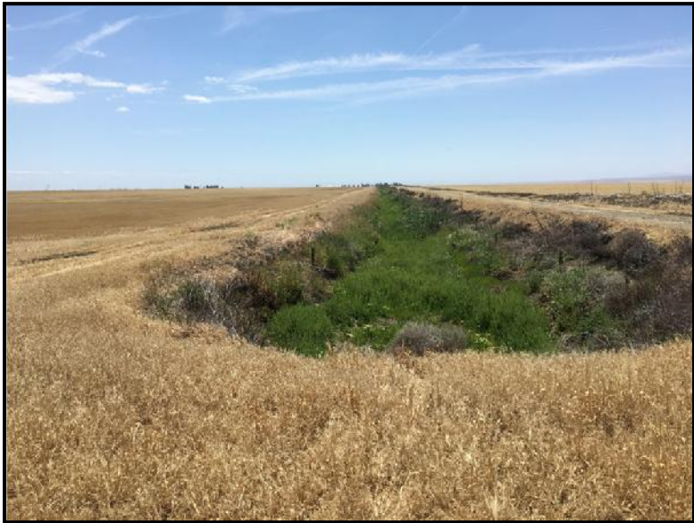
Unlined canal on Site facing south
