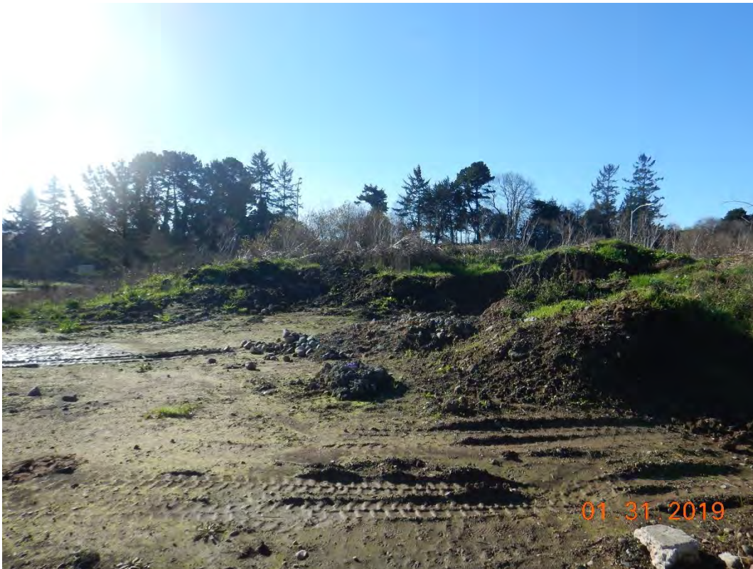
Photo 4. Looking southwest towards temporary soil storage pile from adjacent construction.
