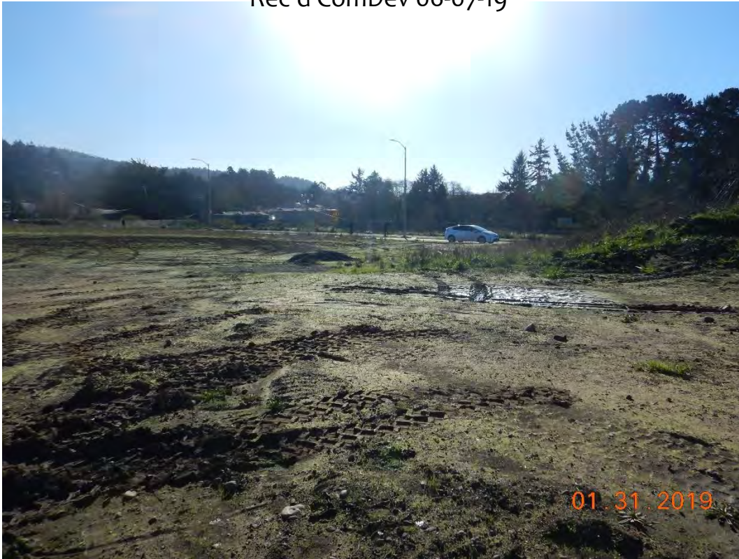
Photo 5. Looking south across heavily compacted area.
