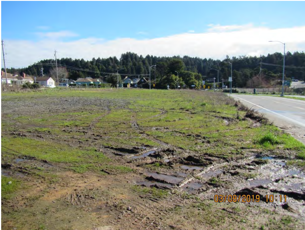
Photo 19. Looking east across southern portion of compacted fill area.
