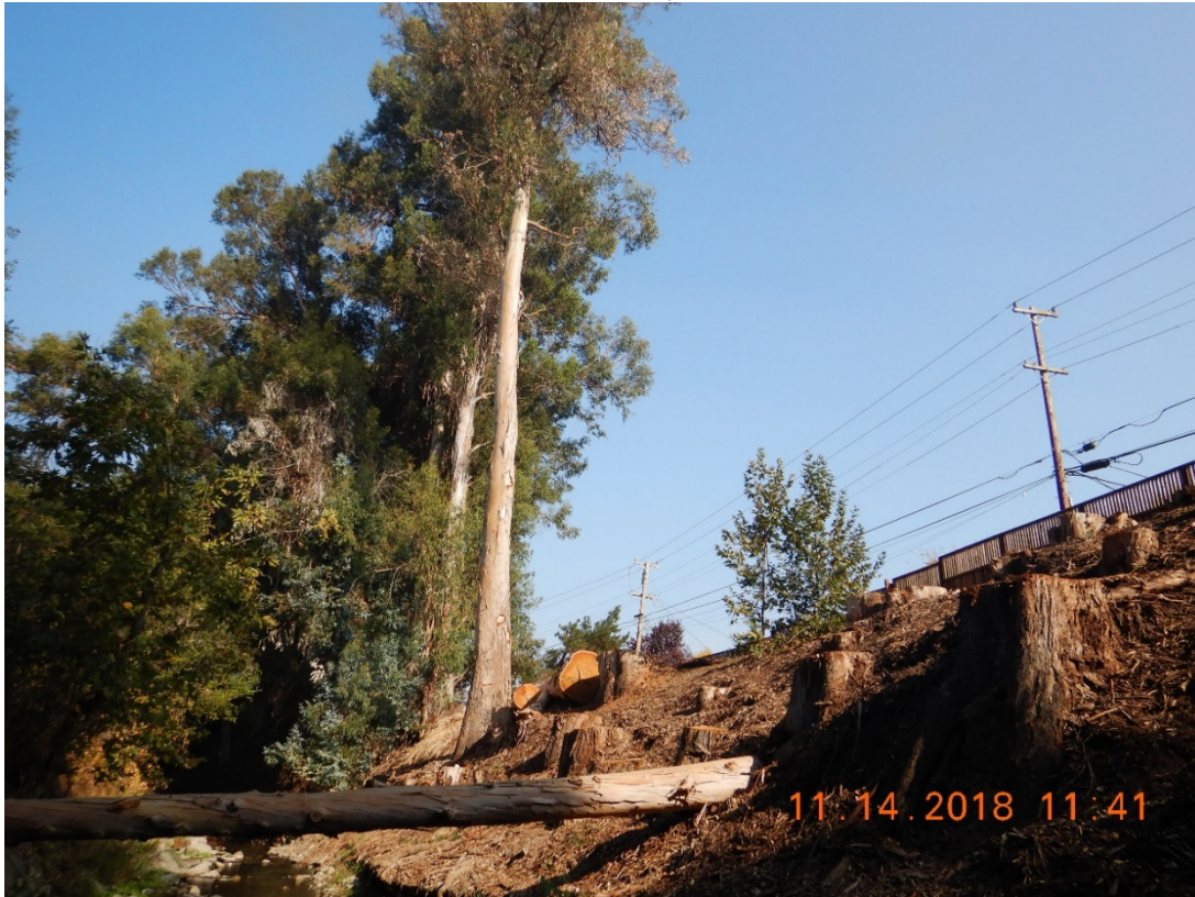
Photo 1: Foreground showing tree removal completed earlier in 2018.
