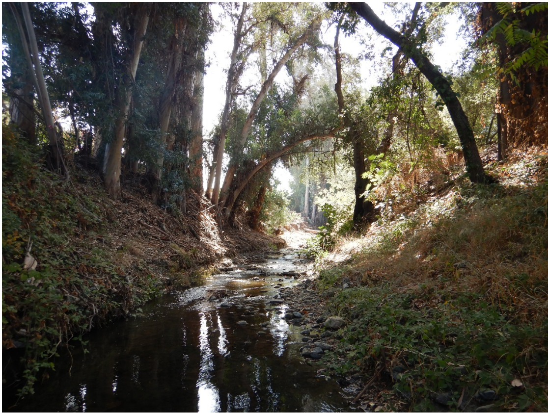
Photo 5: Photo showing several leaning hazard trees on the left bank; 9/27/18
