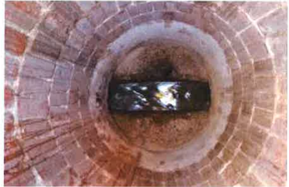
Manhole Before Install
