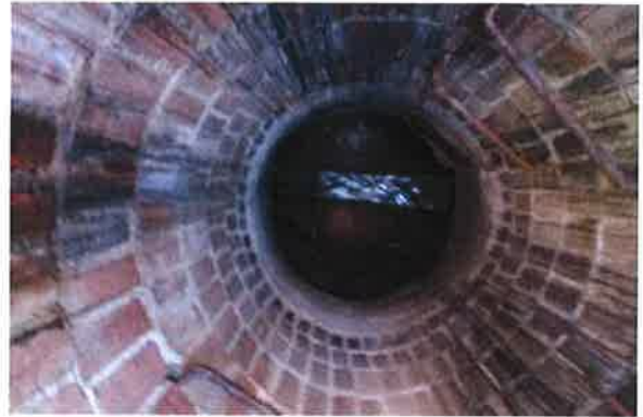
Manhole Before Install
