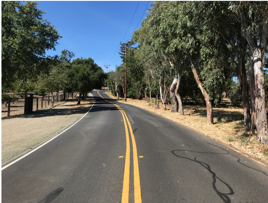
7. View of Taaffe Road looking west (uphill) just west of Elmberg Ridge Road
