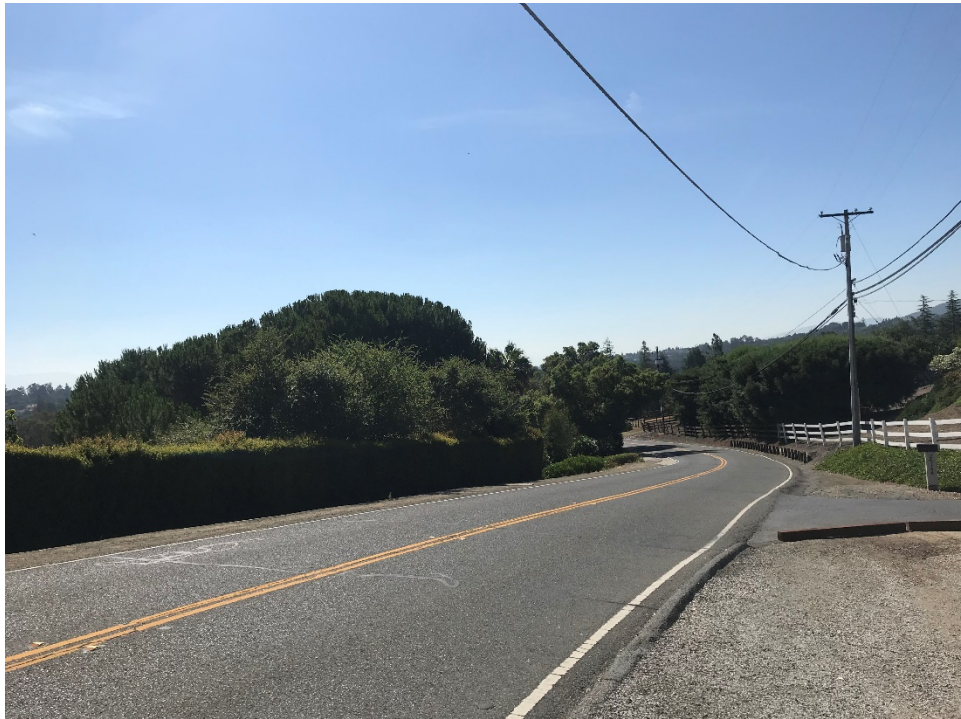
10. View of Elena Road looking southeast from Taaffe Road intersection
