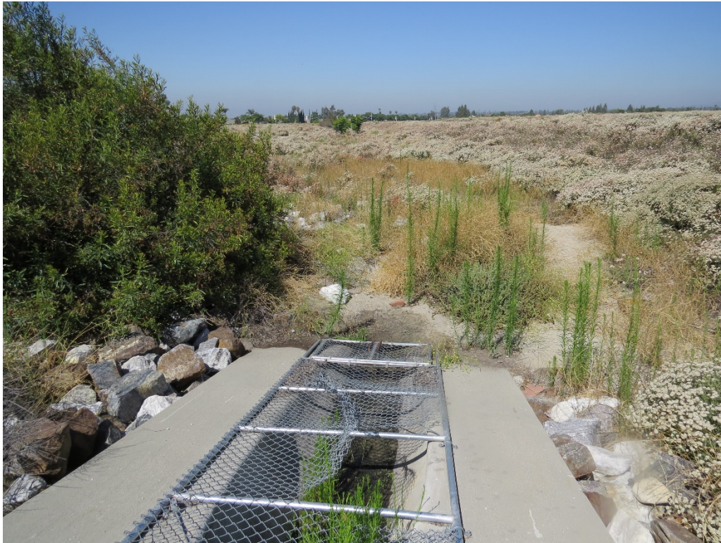
Photograph 9: Looking west over the outflowing culvert.
