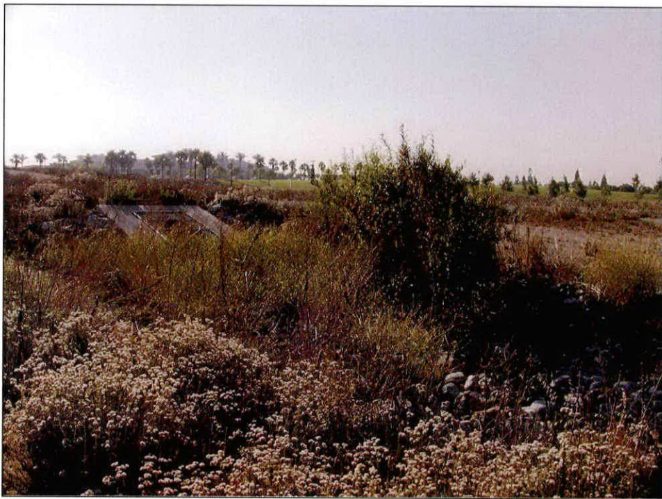
PHOTOGRAPH 8: View of culvert in the center of the site as seen facing southeast. Showing mule fat and California buckwheat.
