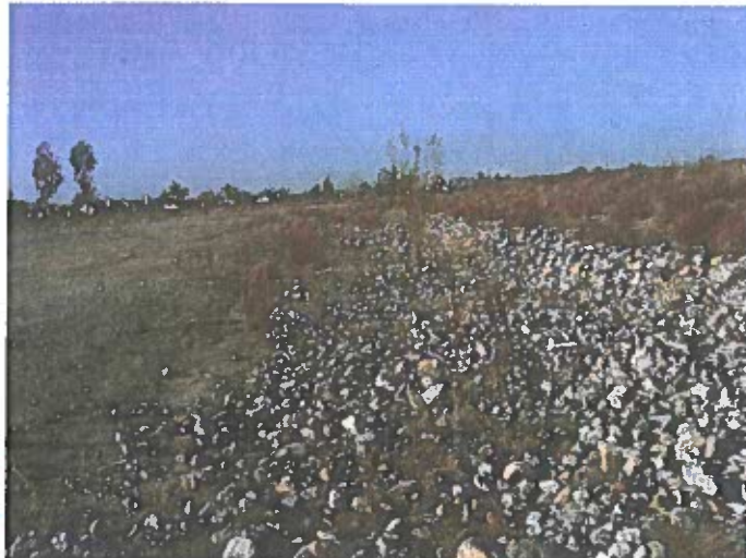
Photo 2: Channelized portion of Drainage A, lined with imported cobble and river-rock looking southwest.
