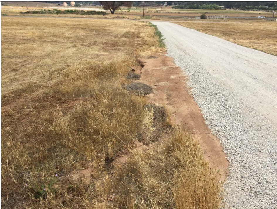
Photo 8: Erosional rill terminus, approximately 100 feet in length before turning into sheet flow, west of unnamed gravel, facing north.
