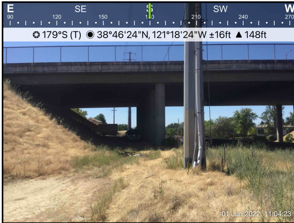
Photo 1. Overpass near Staging Area
