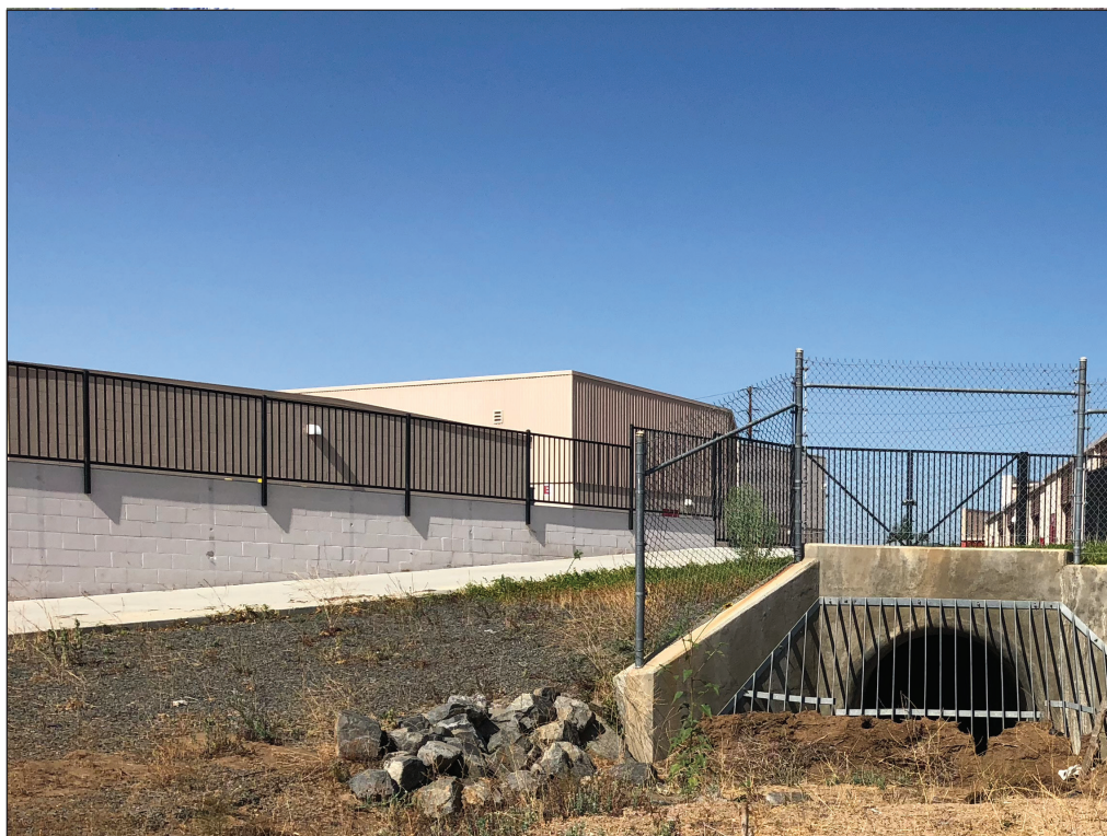
Photo 6. Culvert with headwall where drainage terminates. Facing southwest (downstream).
