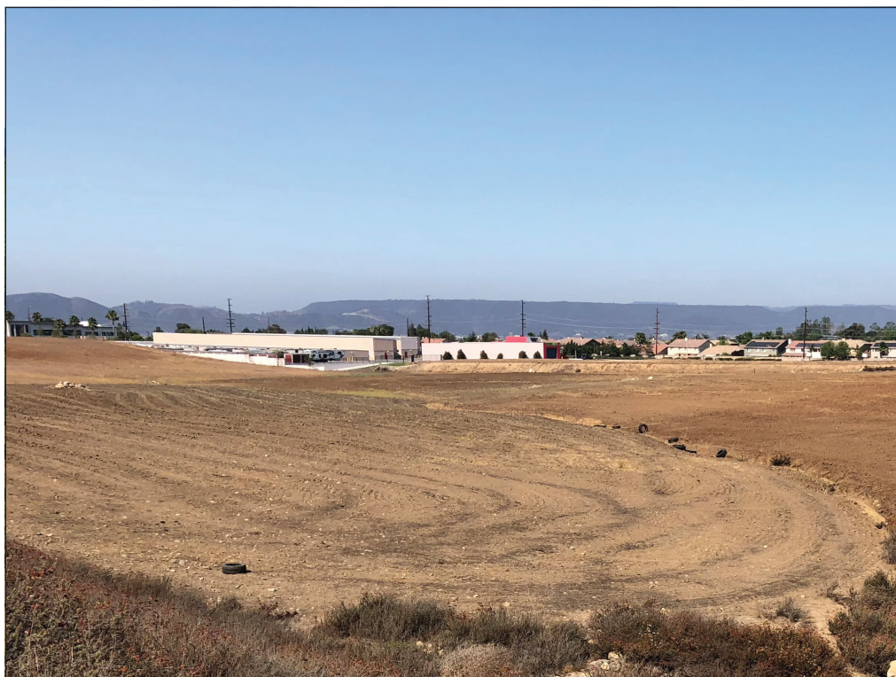
Photo 7. Off-site upstream portion of disturbed drainage where it exits an existing culvert under Sky Canyon Drive and flows southwest towards the study area.
