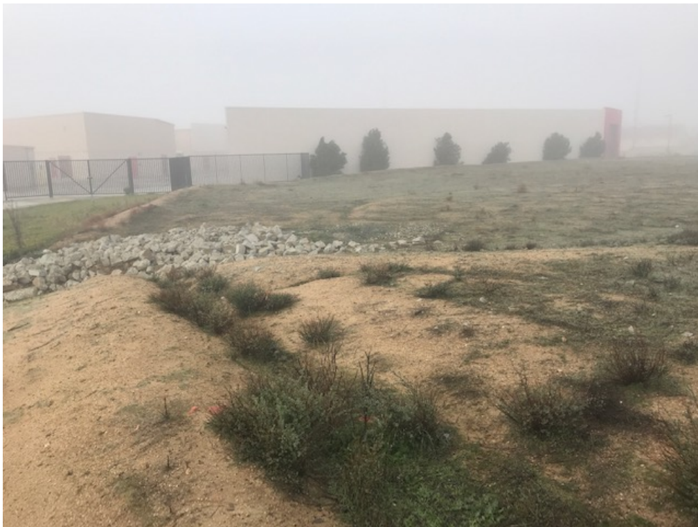
Plate 4. Alternative alignment, 1C with constructed drainage and building. View to the south.
