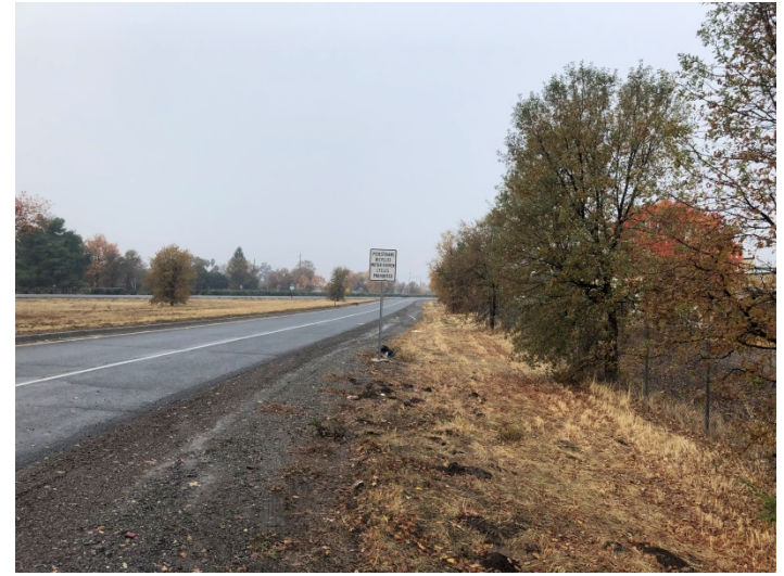
Photo 6. View of SR99 northbound on-ramp from Eaton Road. (November 2019).
