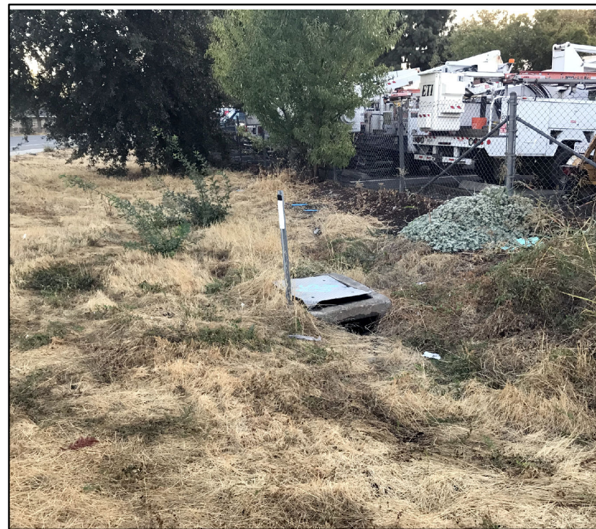
Photo 11: Storm drain at SW corner of Eaton Road and SR 99 offramp.
