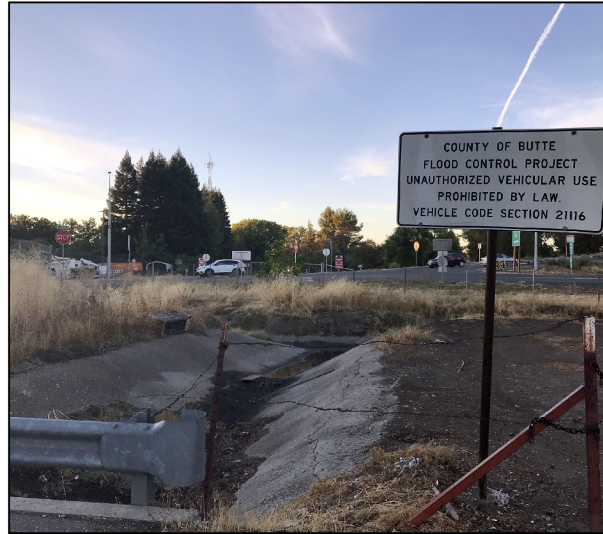
Photo 2: Concrete lined portion of flood control channel.
