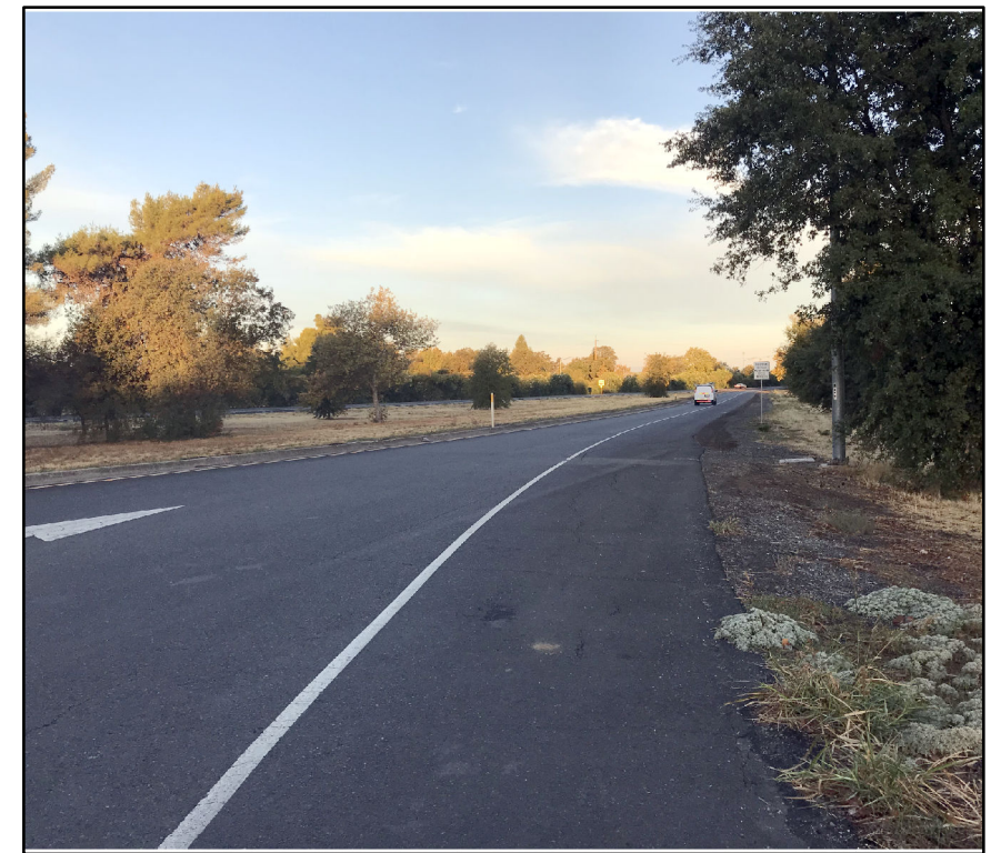
Photo 6: Looking north along SR 99 onramp.
