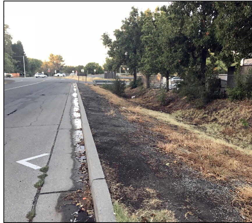
Photo 8: Looking south along Hicks Road at flood control drainage.
