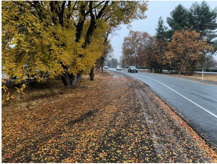
Photo 5. View of SR99 northbound off-ramp to Eaton Road. (November 2019).
