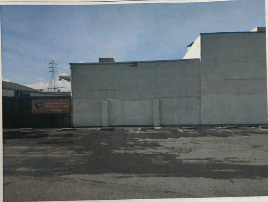
Expansion addition at south end of retail store, viewed facing west.
