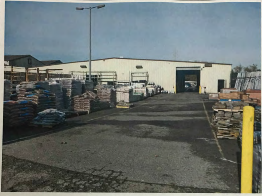
South façade of warehouse and pick-up drive-thru, viewed facing northwest.
