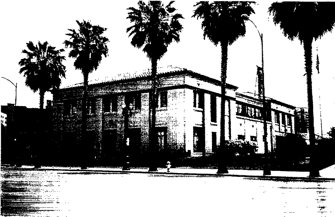
Photo 1: Main Office - View from NW
