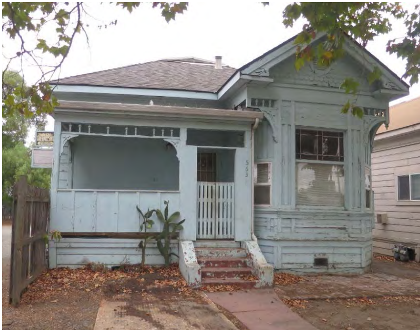
P5b. Description of Photo: South (front) façade, view northwest (September 18, 2019)
