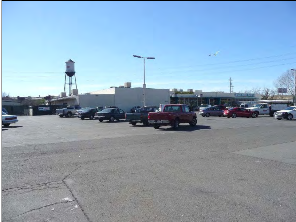
Photograph 2. Main store building, camera facing northwest
