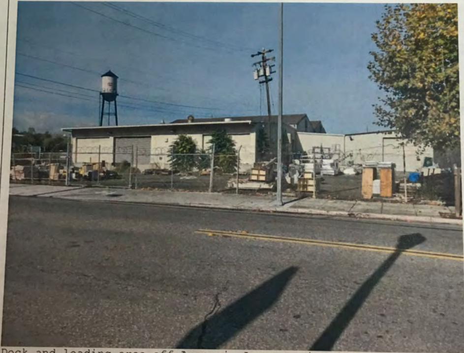
Dock and loading area off Auzerais Avenue, viewed facing northwest.
