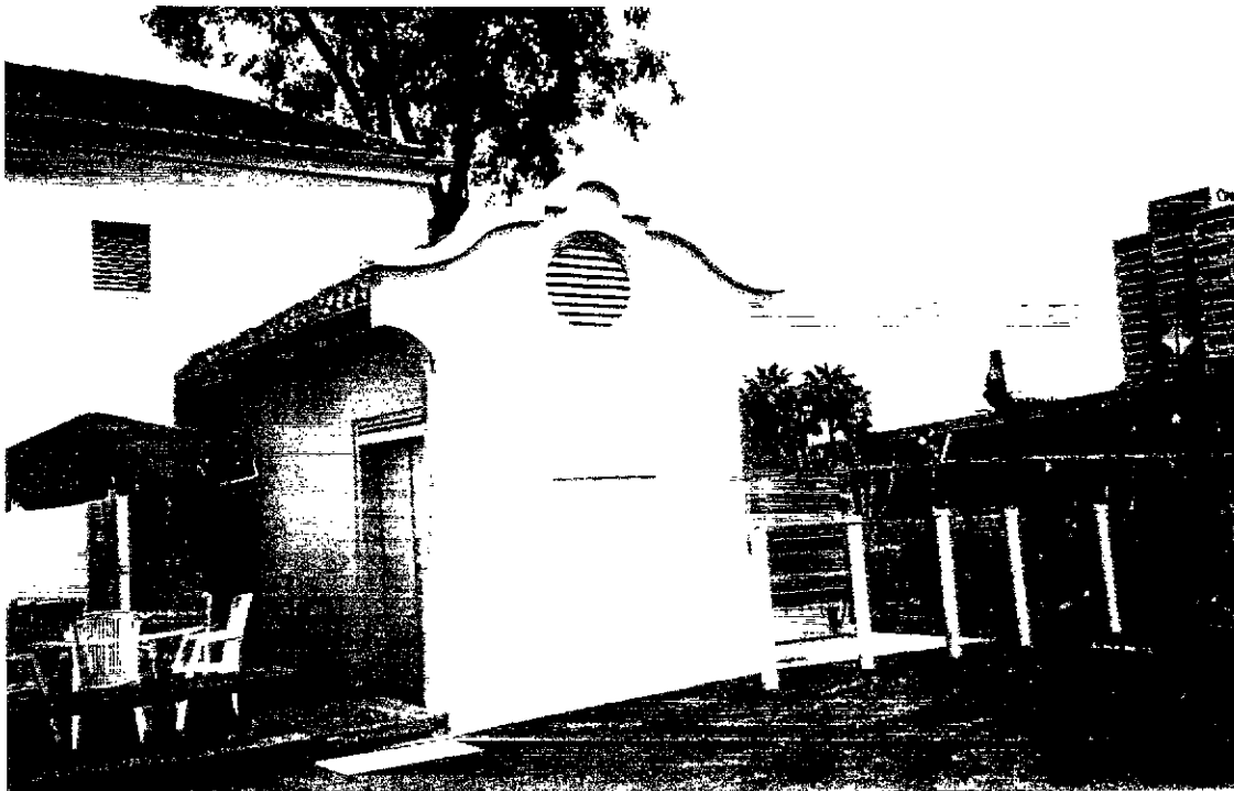
Photo 6: Transformer House - View from SW
