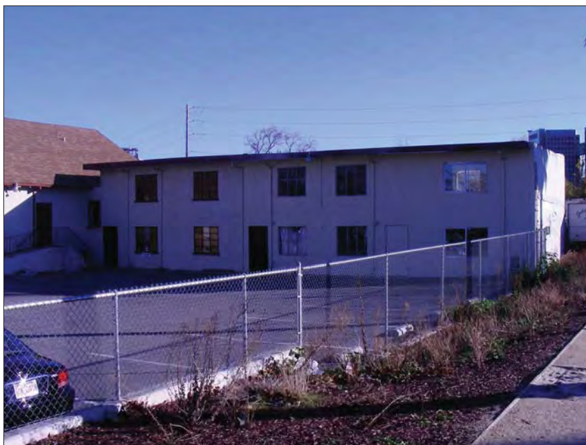
Photograph 3: Education wing, camera facing northeast, December 11, 2007.
