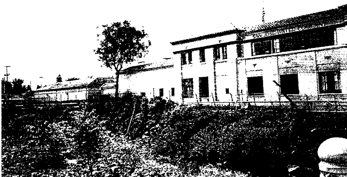
Photo 4: Power House and Related Buildings - View from NE
