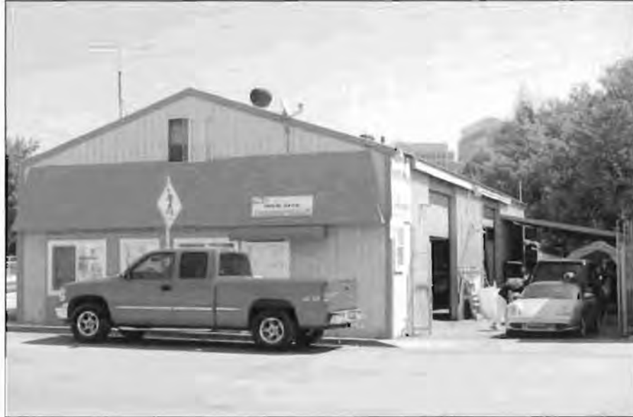
View from the south
