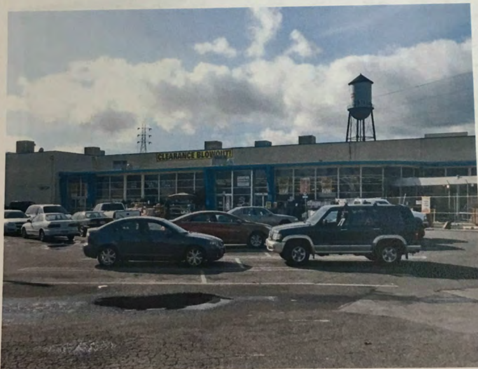
Left side of main entry façade viewed facing southwest.
