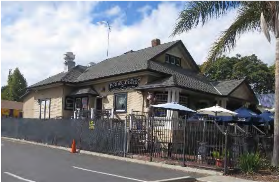
P5b. Description of Photo: East (front) and south façades, view northwest (September 18, 2019)
