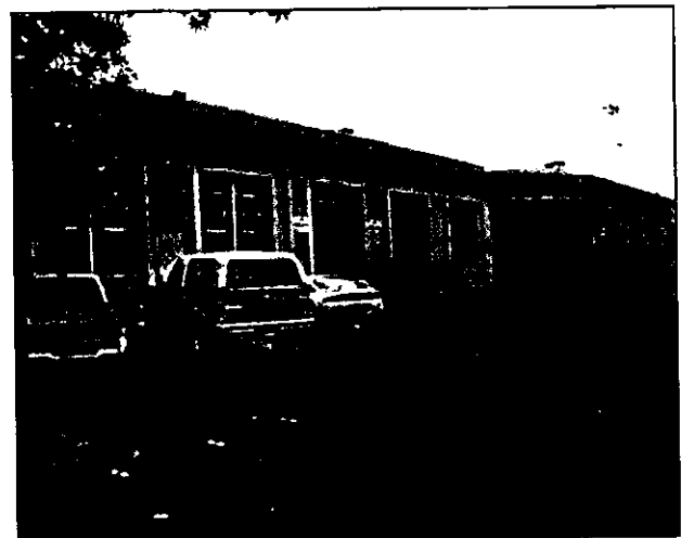
Figure 3. North elevation with addition, towards southwest.
