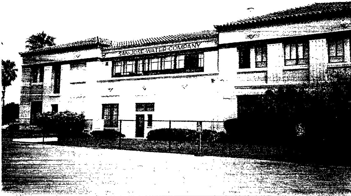
Photo 3: Main Office - View from SW
