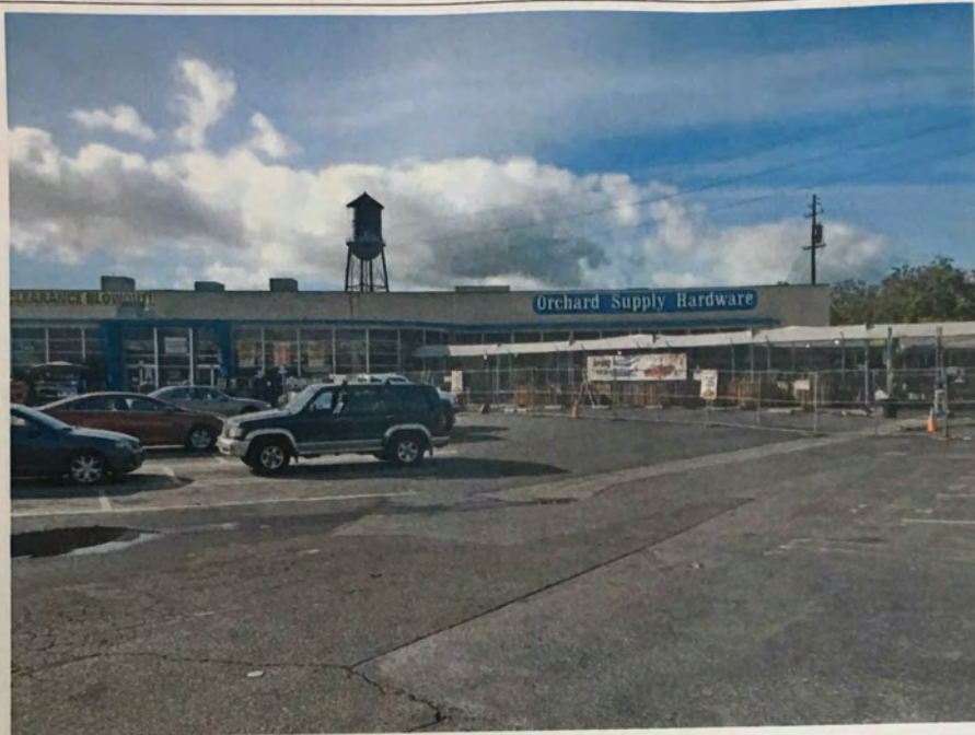
Right side of main entry façade, viewed facing west.
