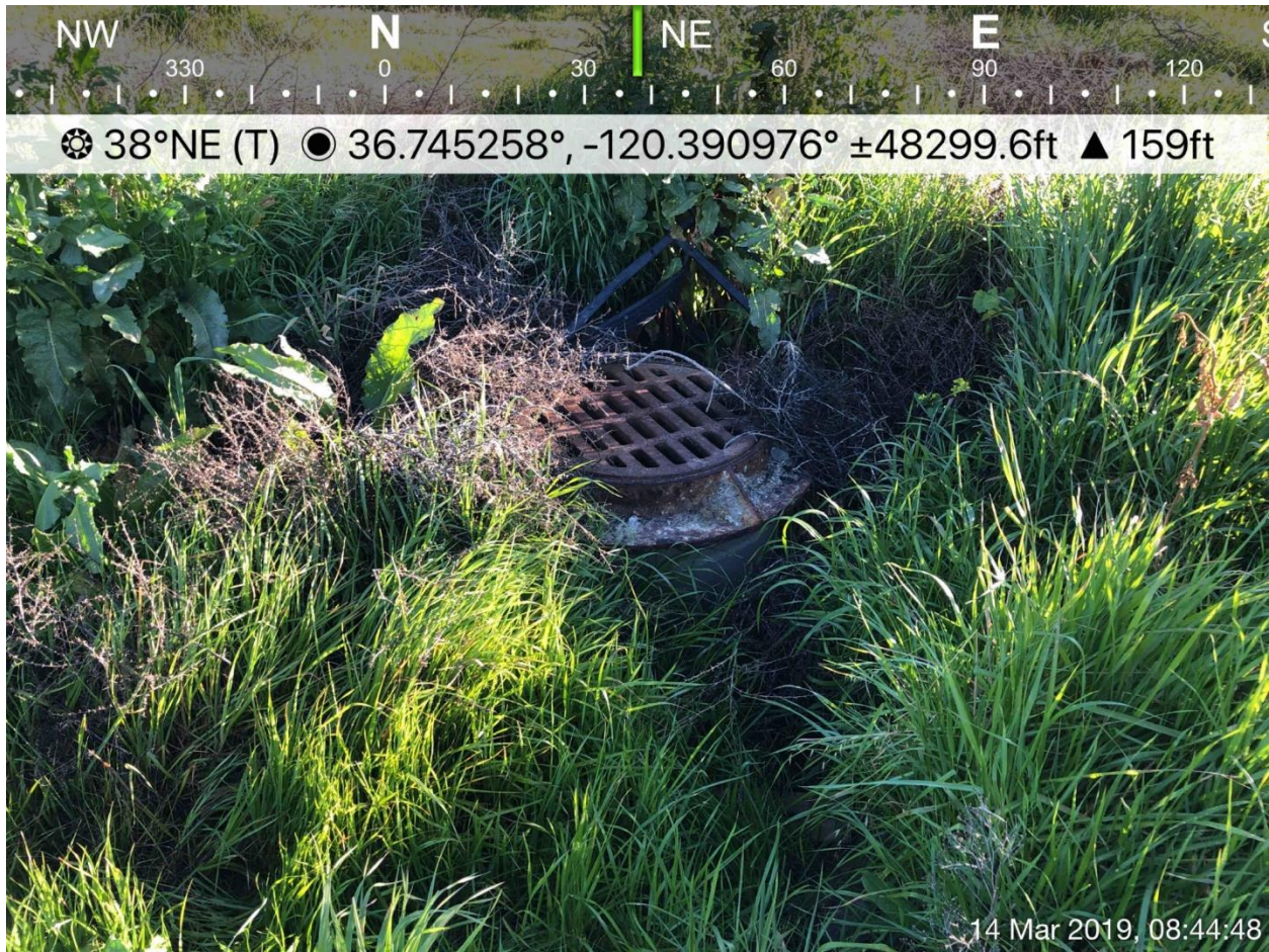
Photograph 5: Drainage outlet structure near the northeast corner of the ruderal lot.
